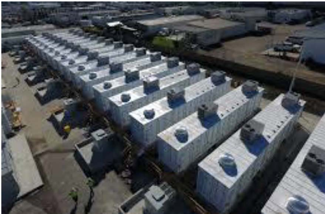
FIGURE 2.0-13 BATTERY ENERGY STORAGE SYSTEM CONTAINERS
