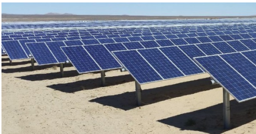
Typical Single-Axis Tracking Solar Panels
