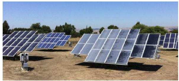
Typical Dual-Axis Tracking Solar Panels
