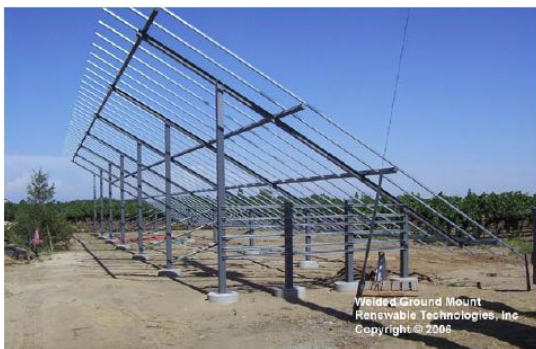
Typical Fixed-Tilt Mounting Structure
