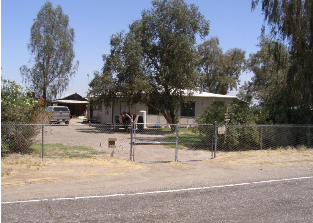
Figure 28. 1596 Fisher Road, Buildings 1 and 3c.
