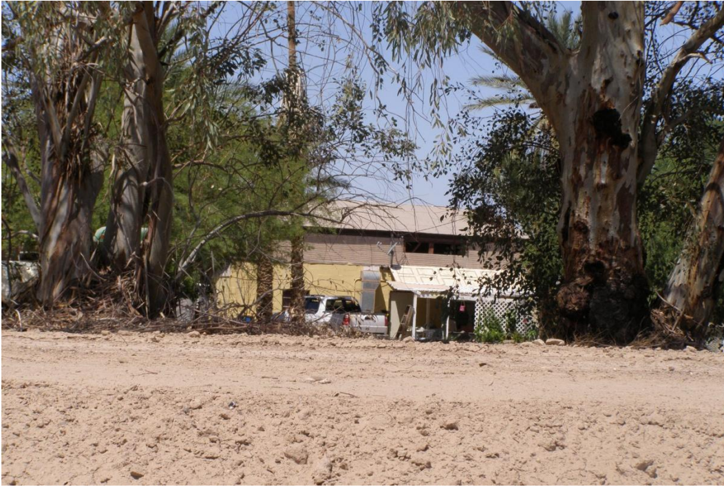
Figure 16. Brockman Ranch, Building 3.
