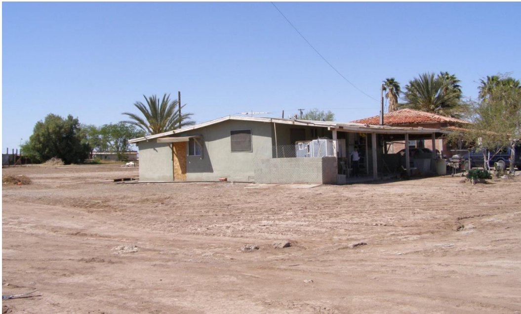
Figure 11. Mount Signal, Building 4.
