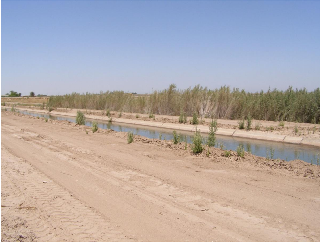
Figure 5. Westside Main Canal.
