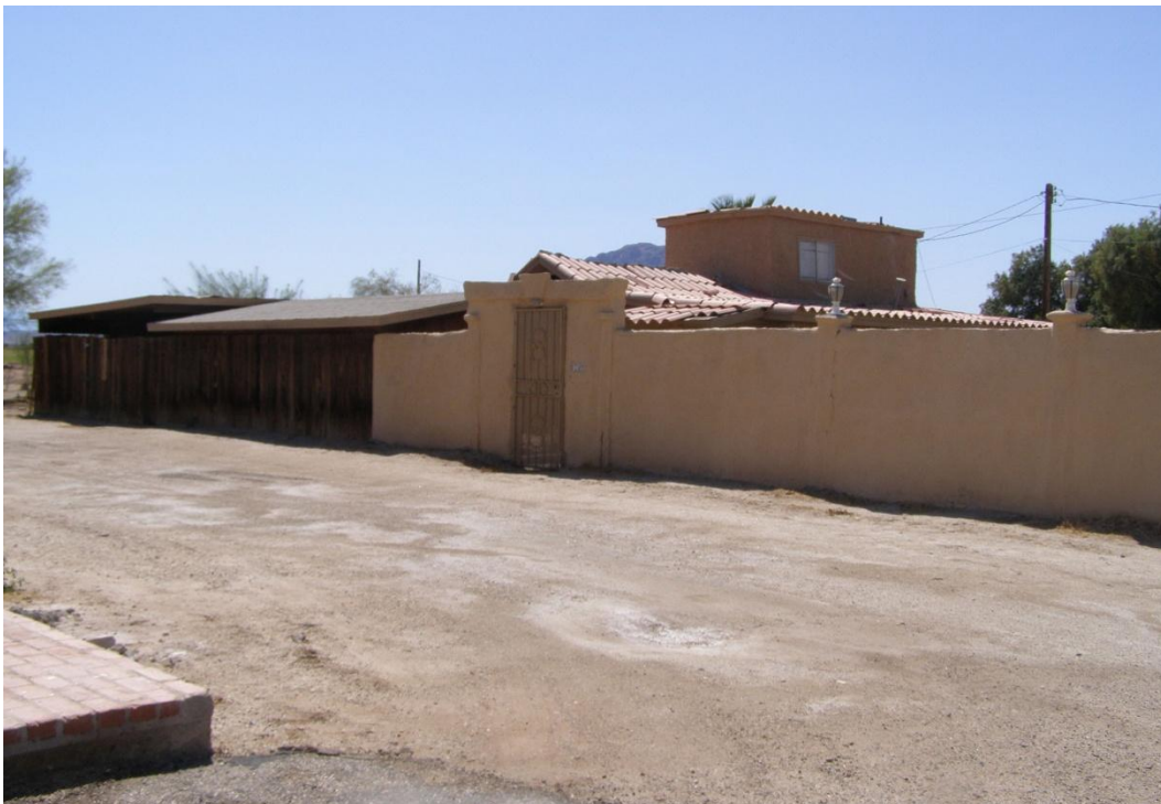
Figure 9. Mount Signal, Buildings 2a and 2b.
