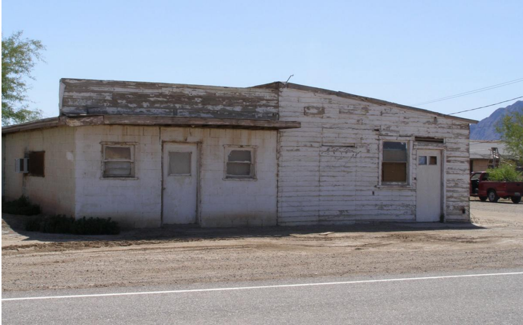
Figure 12. Mount Signal, Building 5.
