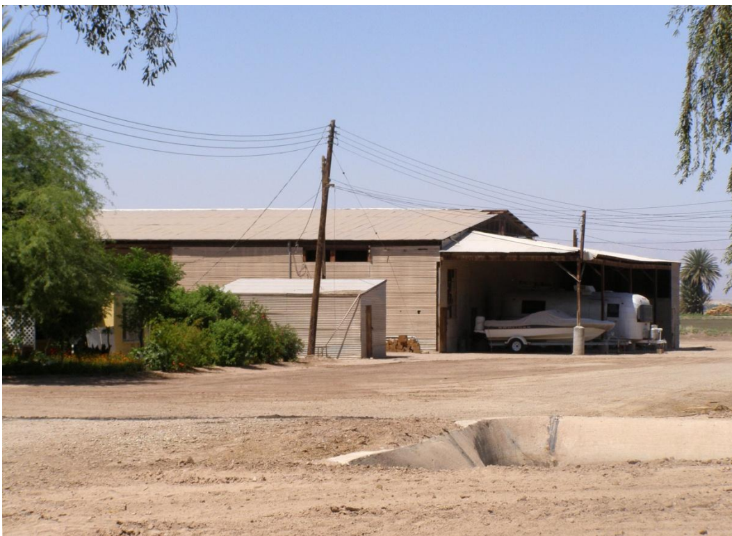
Figure 15. Brockman Ranch, Building 2.
