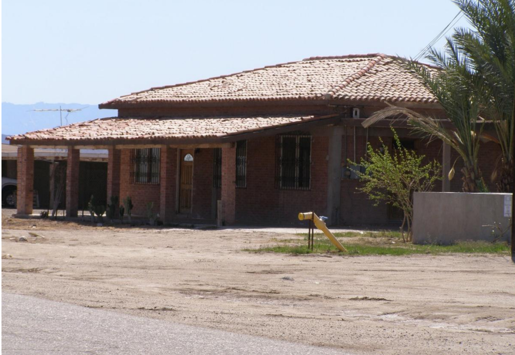
Figure 10. Mount Signal, Building 3.
