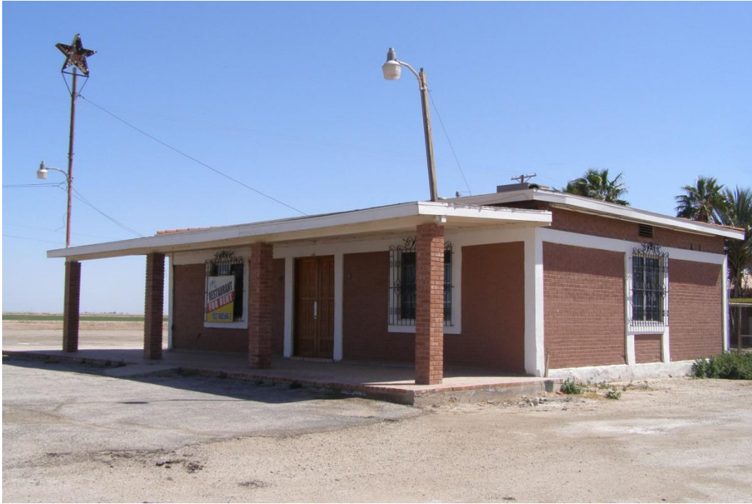
Figure 8. Mount Signal, Building 1.
