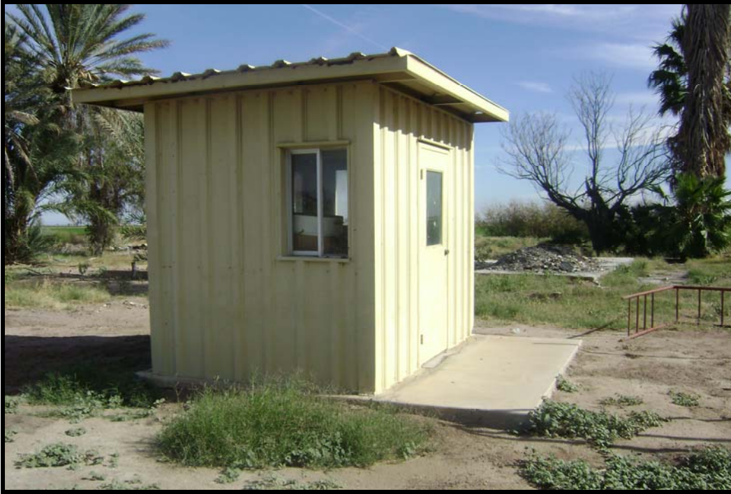
Photo 17: One of two storage sheds in Parcel 4.
