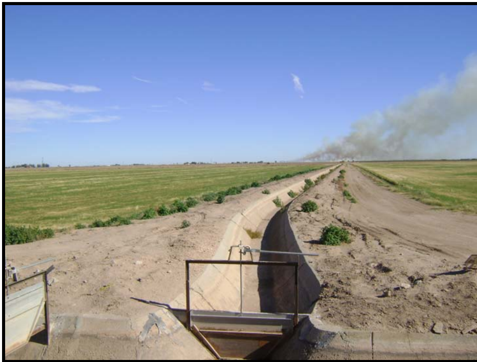
Photo 6: Looking east along the southern boundary of Parcel 2.
