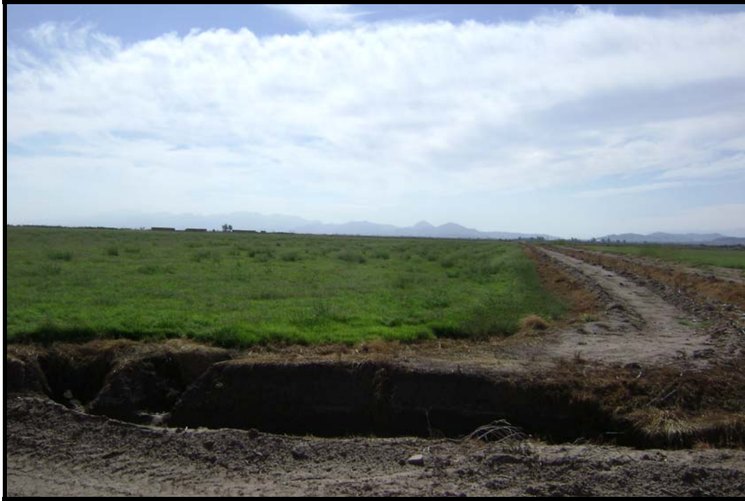
Photo 7: Looking south along the western boundary of Parcel 3.
