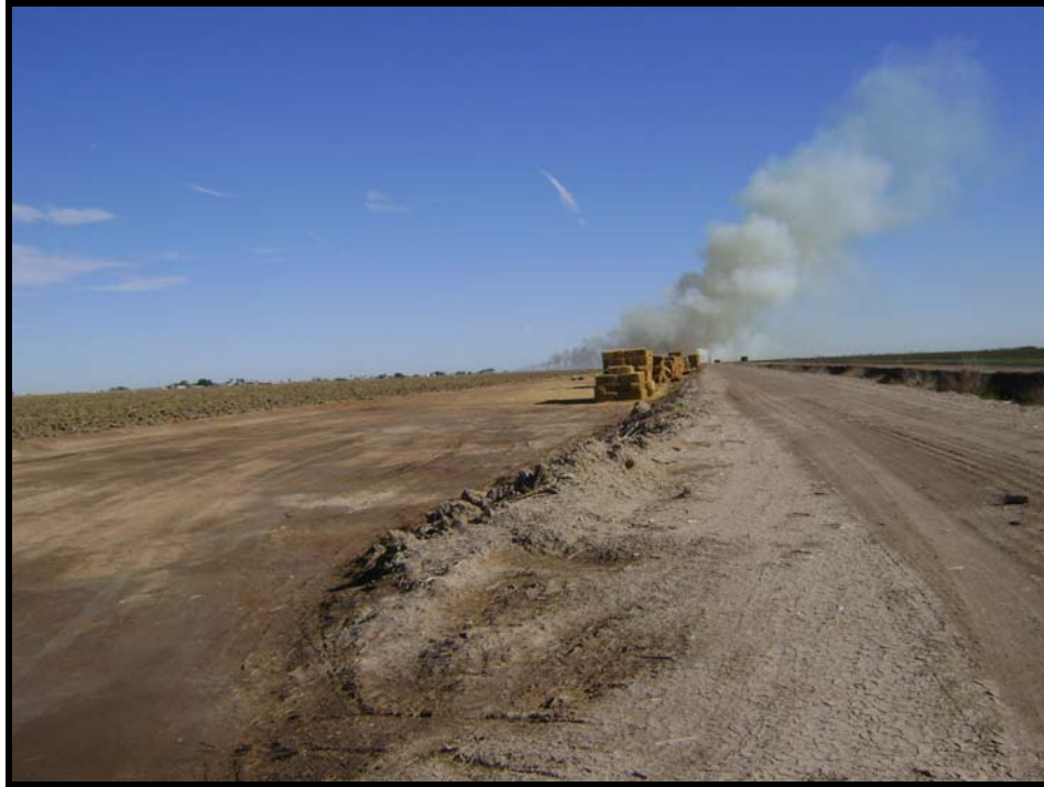
Photo 9: Looking east along the southern boundary of Parcel 3.
