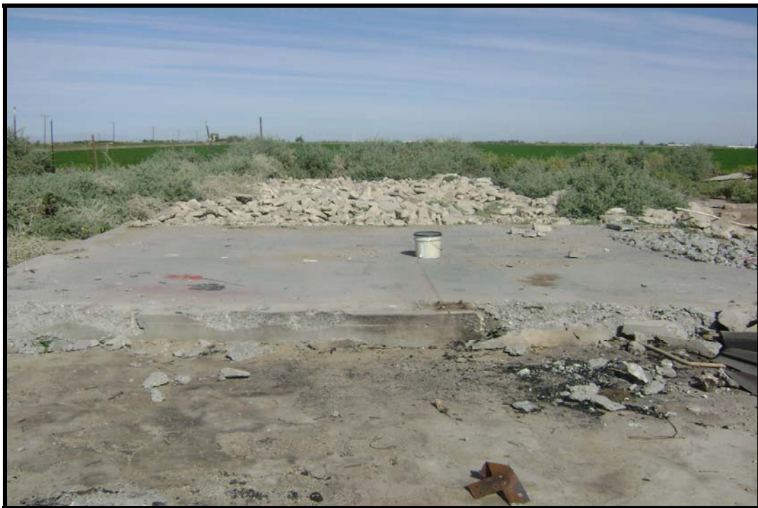
Photo 14: Concrete slab and rubble in the central northern area of Parcel 4.
