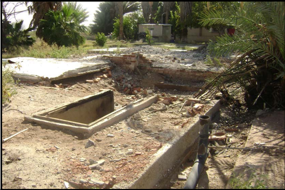
Photo 15: Old foundation of brick building in the central eastern area of Parcel 4.
