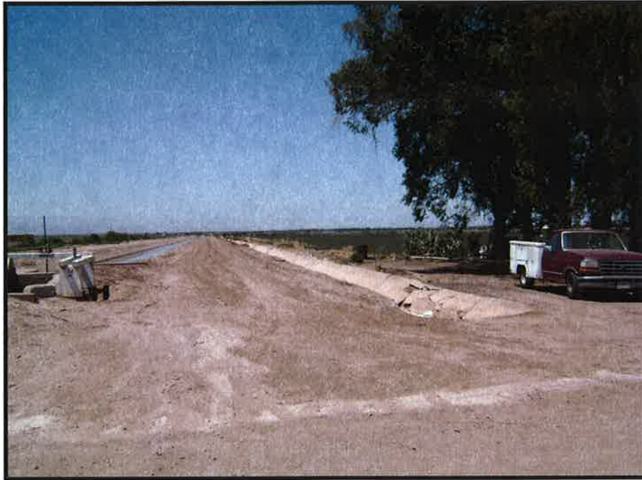
Photo 5: Looking west along the southern boundary of section 3.
