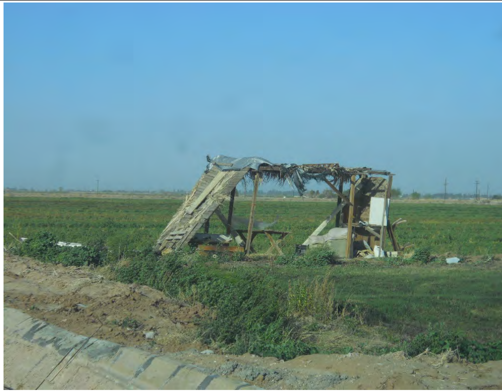
Photograph 15 Comments: APN: 051-350-14 View facing northwest toward shade/shelter structure in central portion of property.
