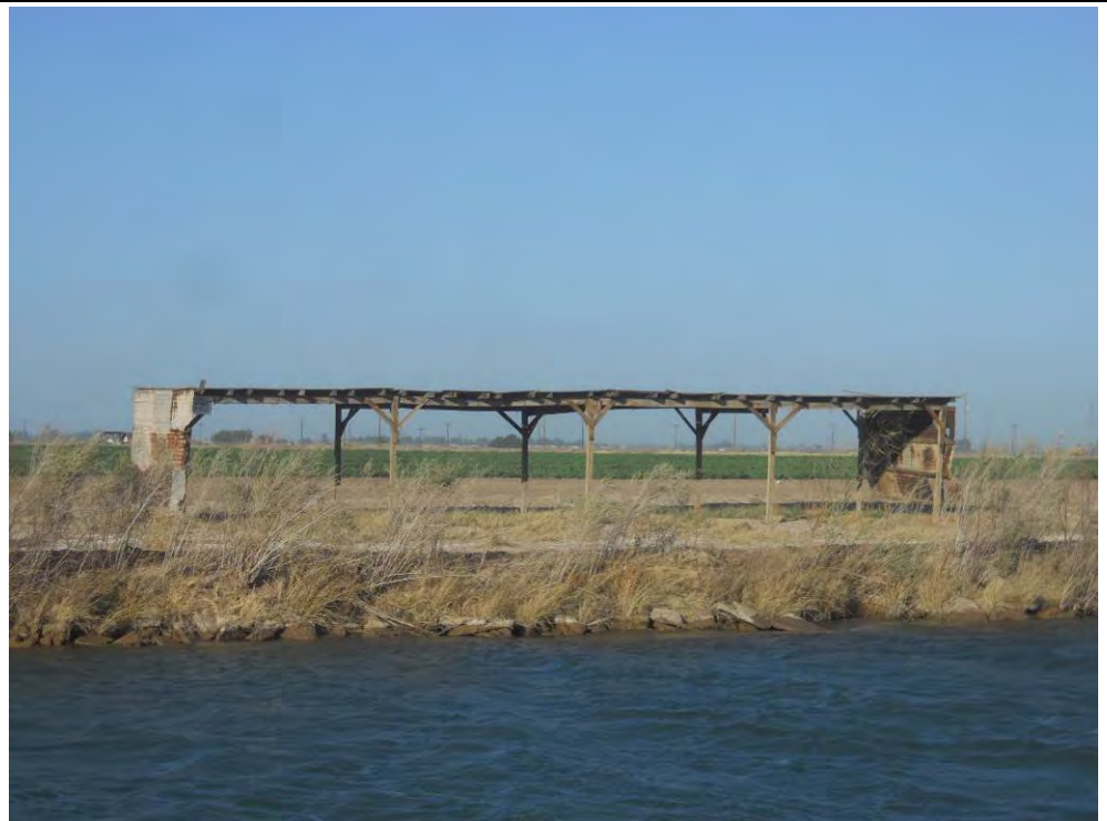
Photograph 16 Comments: APN: 051-350-14 View facing north of bee box shade structure on southern side of parcel.
