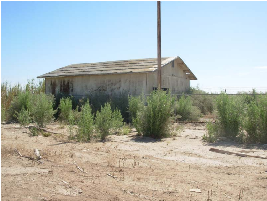
Photo 20. Dilapidated building located on the Childers parcel.
