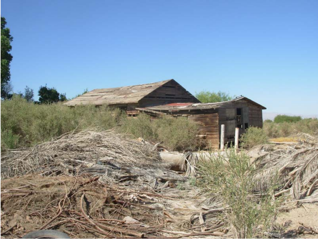
Photo 13. Dilapidated barn located in the eastern portion of Kuhn parcel.
