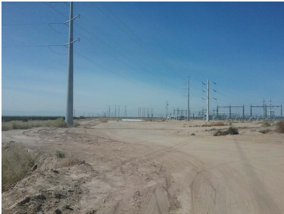
Photo 2: Looking west at the IID substation from the southeast corner of the north parcel.
