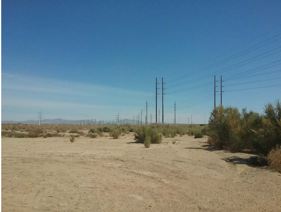
Photo 9: Looking northeast from the southwest corner of the north parcel.
