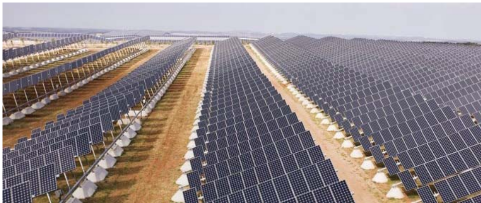
Typical Single-axis Tracking Solar Panel Rows
