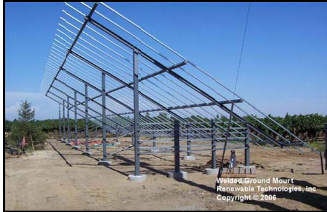
Typical fixed-tilt mounting structure
