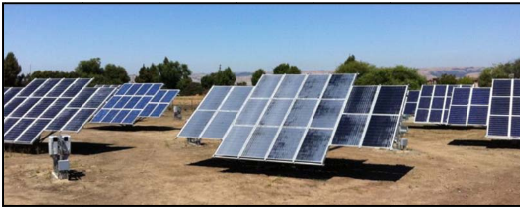
Typical dual-axis tracking solar panels
