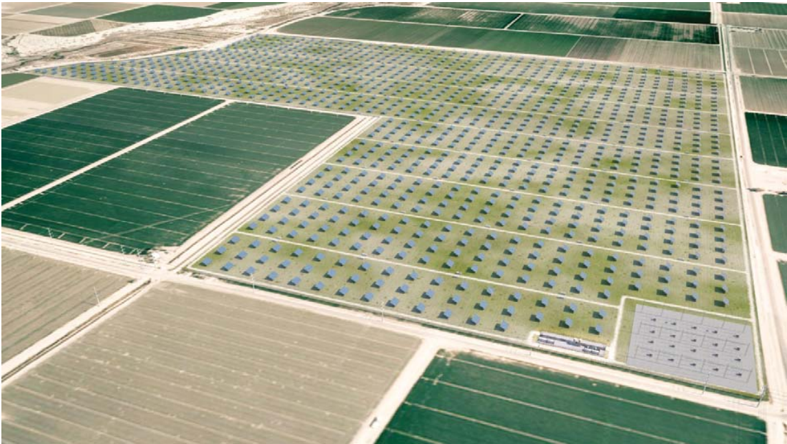
Iris Solar Farm: View from Ferrel Rd (NE corner of 059-120-001), looking SW
