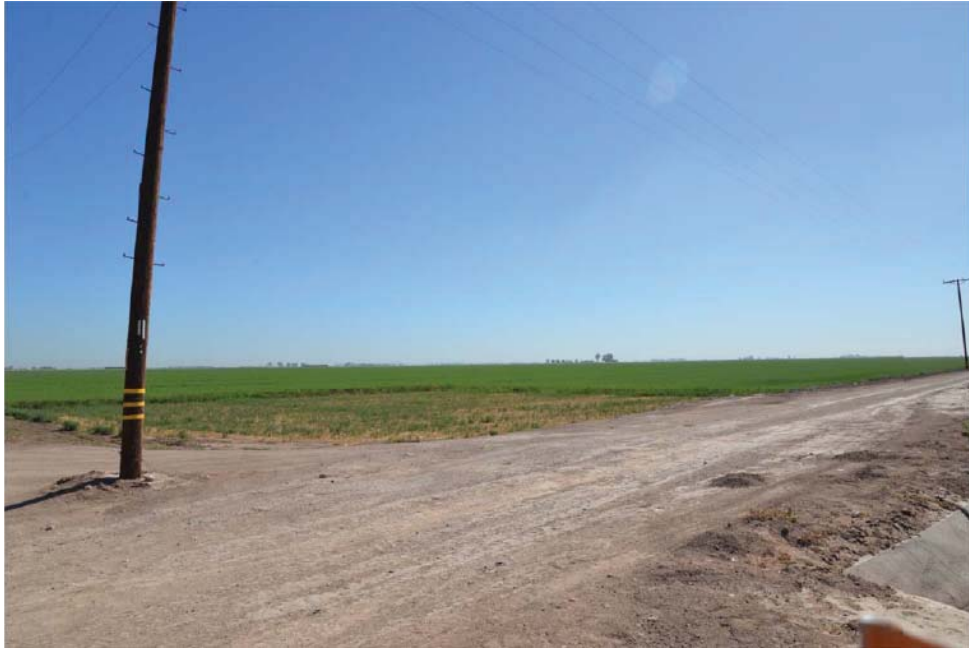
Iris Solar Farm: View from the crossroads between Ferrel Rd and State Route 98 (SW corner of 059-120-001), looking NE, before construction
