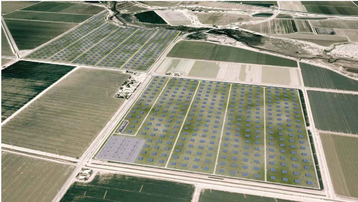
Ferrell Solar Farm: SE corner of 059-050-001, looking NW
