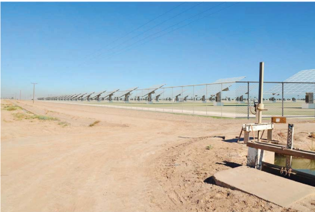
Iris Solar Farm: View from State Route 98 (SE corner of 059-050-003), looking NW, after construction
