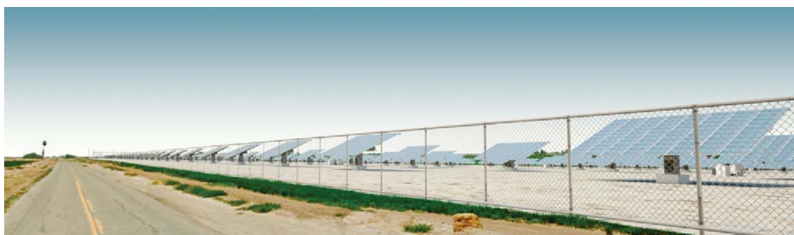
Iris Solar Farm: View from State Route 98 (SE corner of 059-050-003), looking NW, after construction
