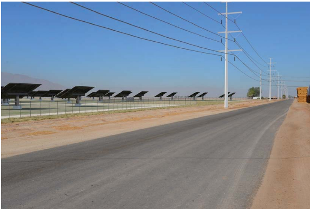
Rockwood Solar Farm: View from Kubler Rd (NW corner of 052-180-048), looking SW, after construction
