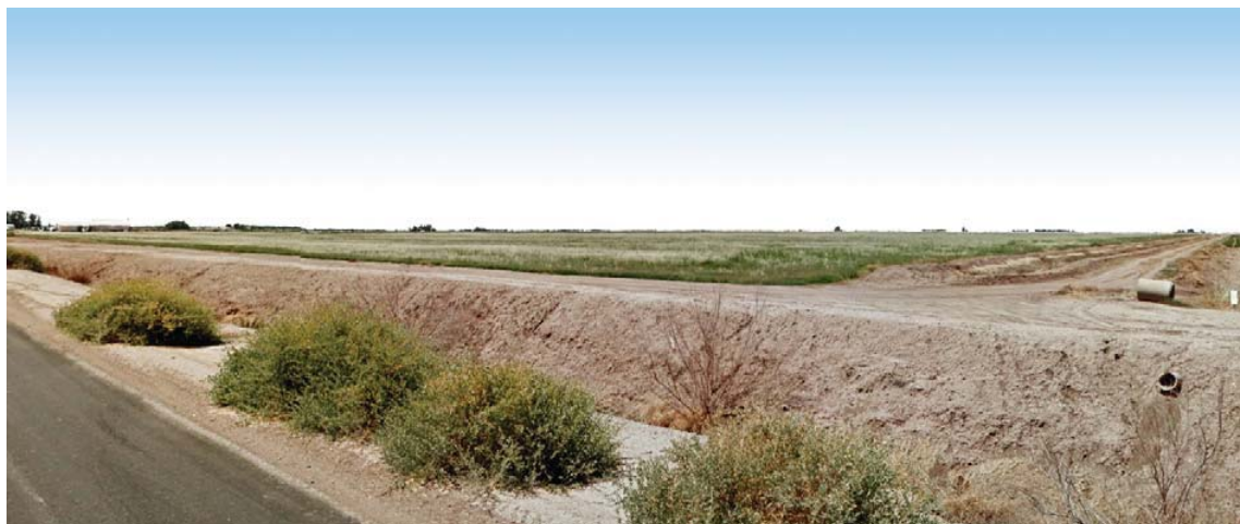
Lyons Solar Farm: View from Kubler Rd (SE corner of 052-180-058), looking NW, before construction
