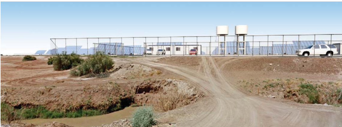
Lyons Solar Farm: View from Kubler Rd (SE corner of 052-180-053), looking NW, after construction
