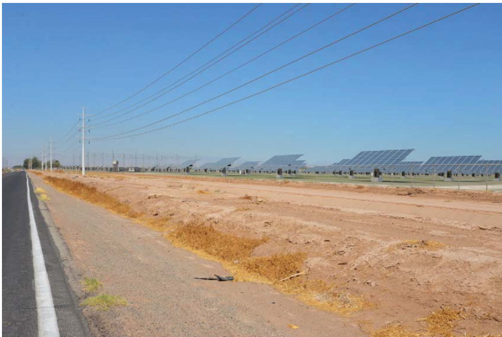
Rockwood Solar Farm: View from State Route 98 (S side of 052-180-064), looking NW, after construction
