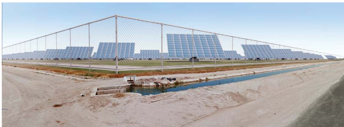
Ferrell Solar Farm: View from Kubler Rd (SW corner of 052-180-042), looking NE, after construction
