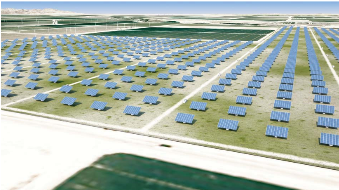
Iris Solar Farm: View from State Route 98 (SE corner of 059-050-003), looking NW
