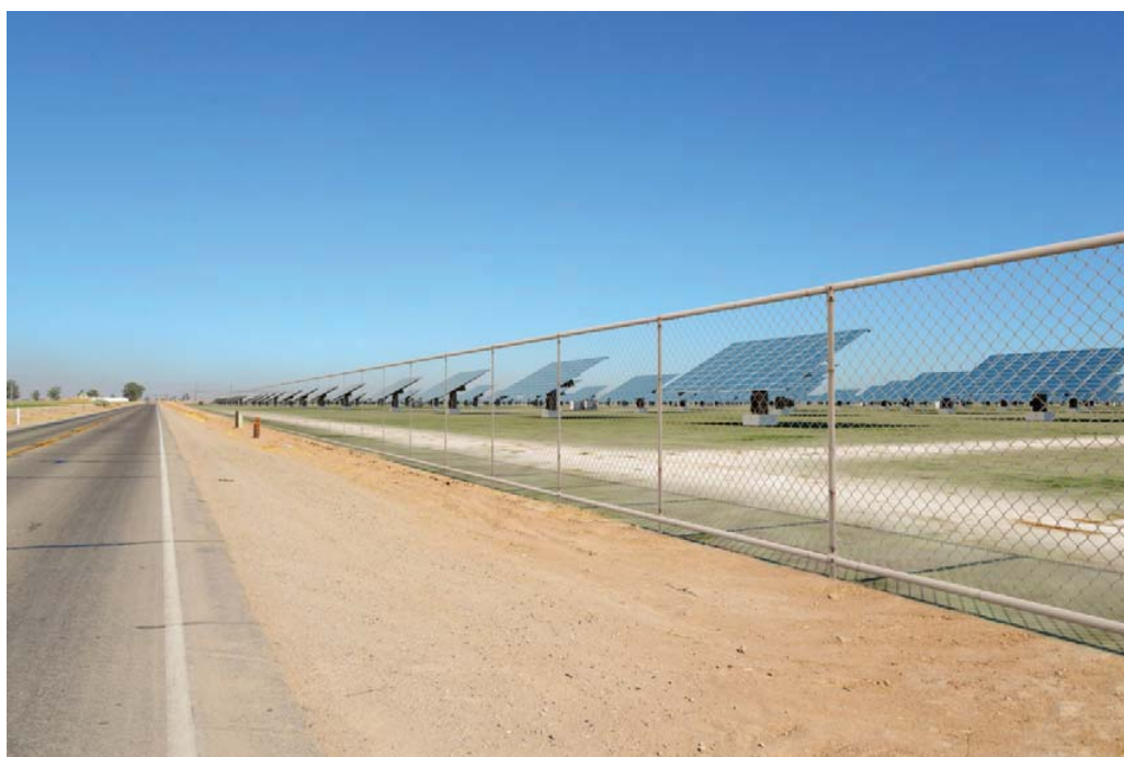
Iris Solar Farm: View from State Route 98 (S side of 059-050-003), looking NW, after construction
