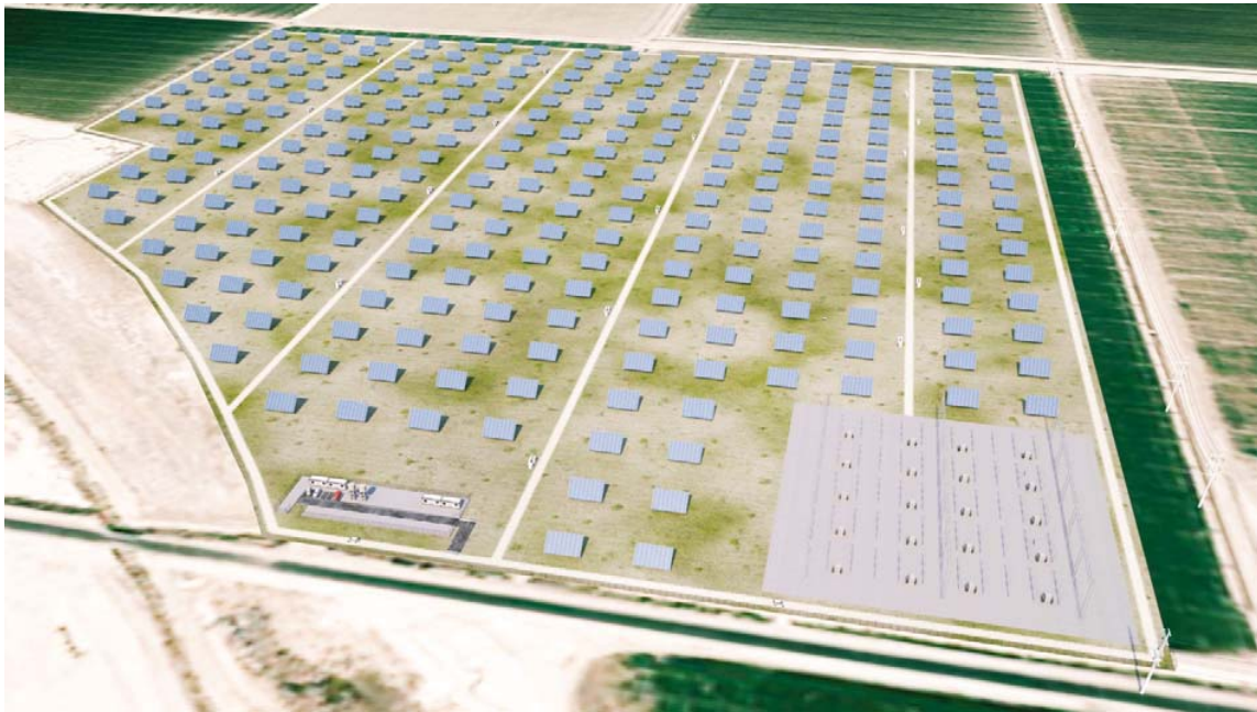
Lyons Solar Farm: View from Kubler Rd (SW corner of 052-180-058), looking NE
