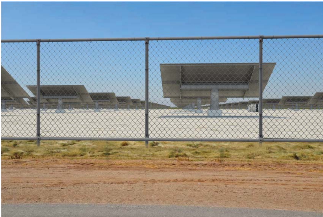
Rockwood Solar Farm: View from Kubler Rd (NW corner of 052-180-048), looking SE, after construction
