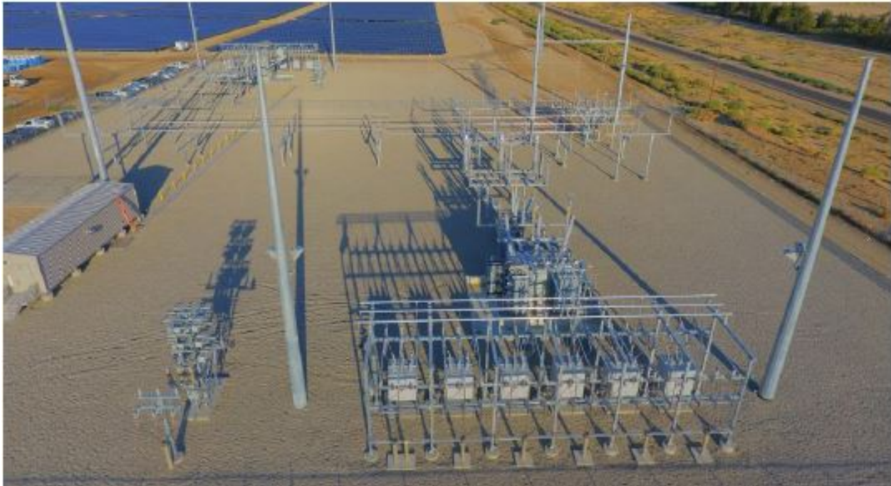
Figure 3-14. Representative Example of Typical Substation Design
