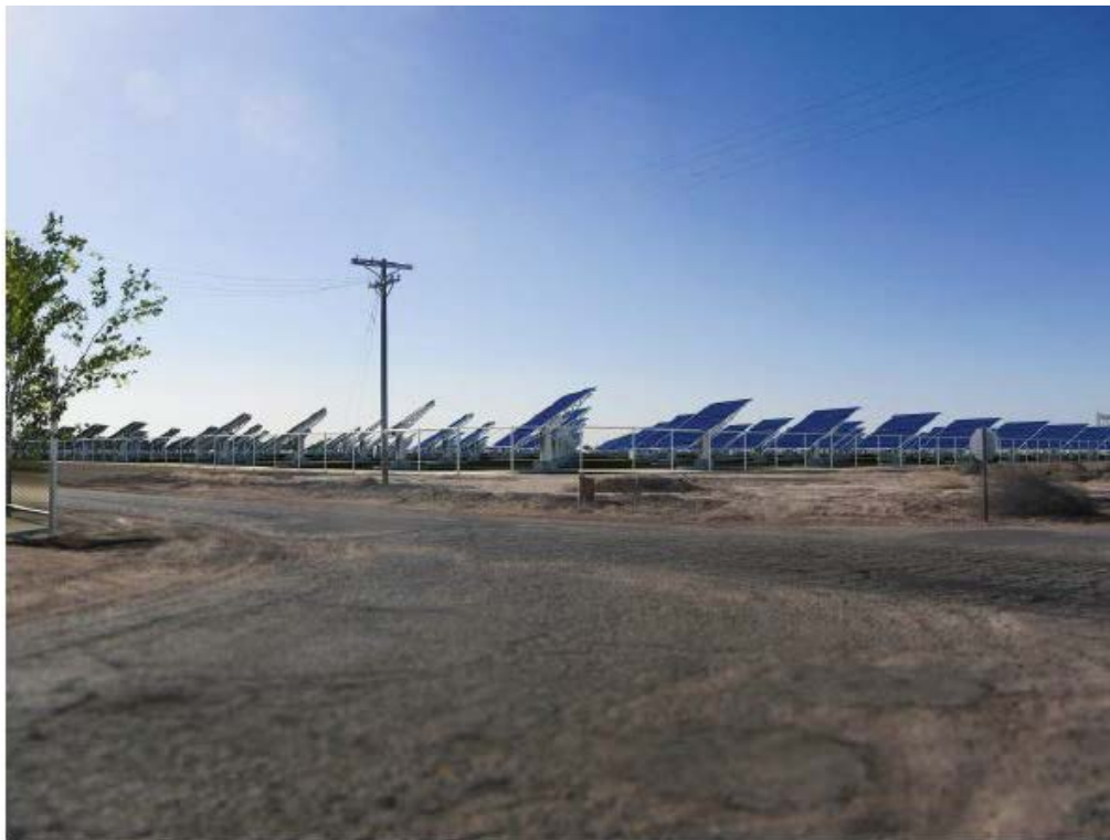
Laurel 4-Solar Farm 1 Proposed Condition: View of solar arrays from the corner of Derrick Road and West Diehl Road facing southeast
