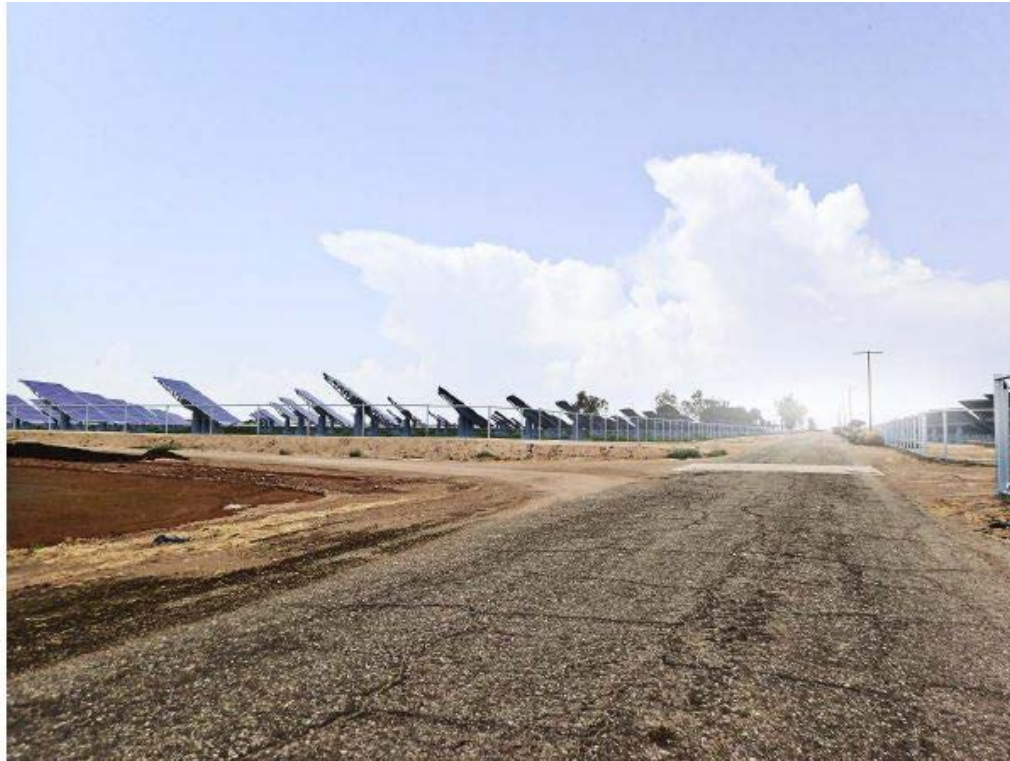
Laurel 3 Solar Farm 3 Proposed Condition: View of solar arrays from the center on West Vaughn Road looking northeast
