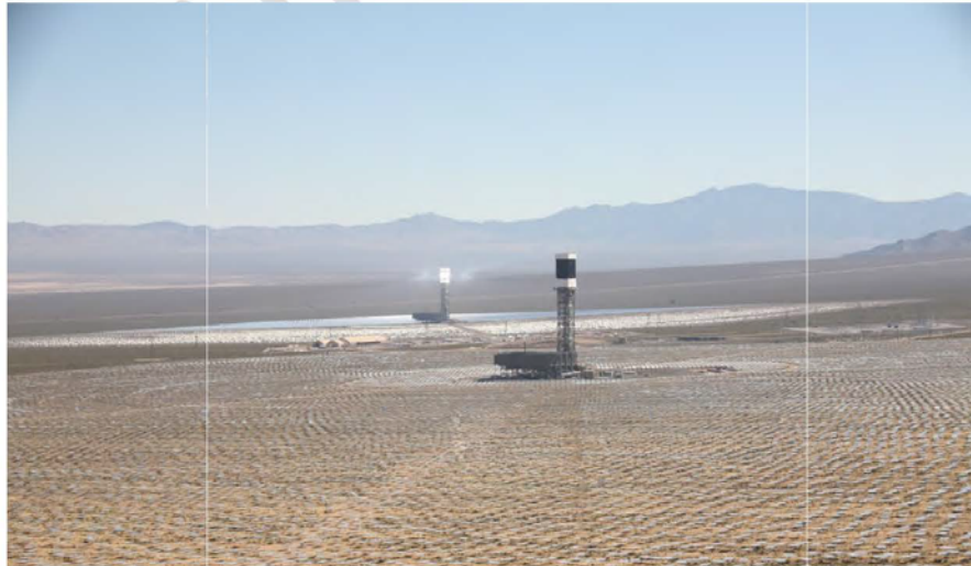
Figure 9: Tower 1 (bright white) is shown under power. Tower 2 (black) is not operating.
