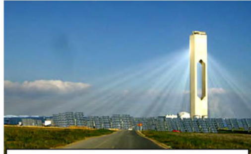
Figure 8: Seville solar power facility ( http://inhabitat.com/sevilles-solar-power-tower )
