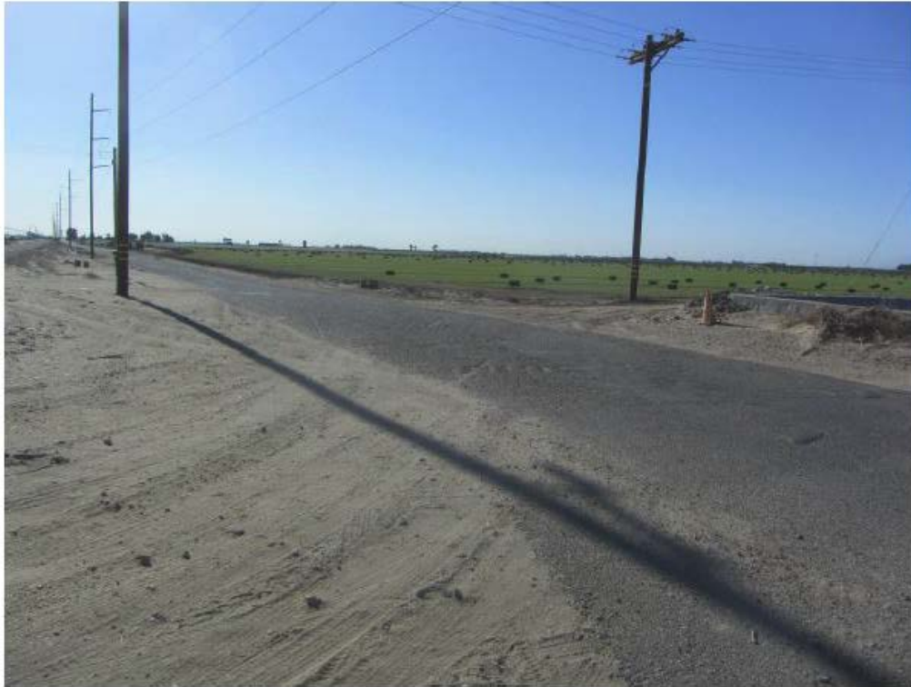
Big Rock Laurel Solar Farm 4 Existing Condition: Corner of Liebert Road and West Wixom Road facing southeast
