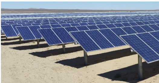
Typical Single-Axis Tracking Solar Panels
