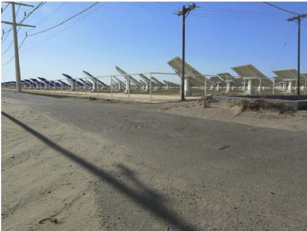
Big Rock Laurel Solar Farm 4 Proposed Condition: View of solar arrays and transmission line from the corner of Liebert Road and West Wixom Road facing southeast
