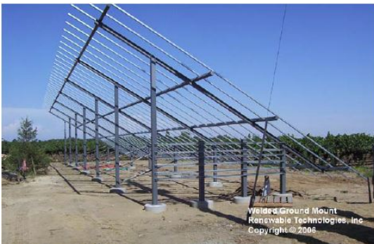
Typical Fixed-Tilt Mounting Structure
