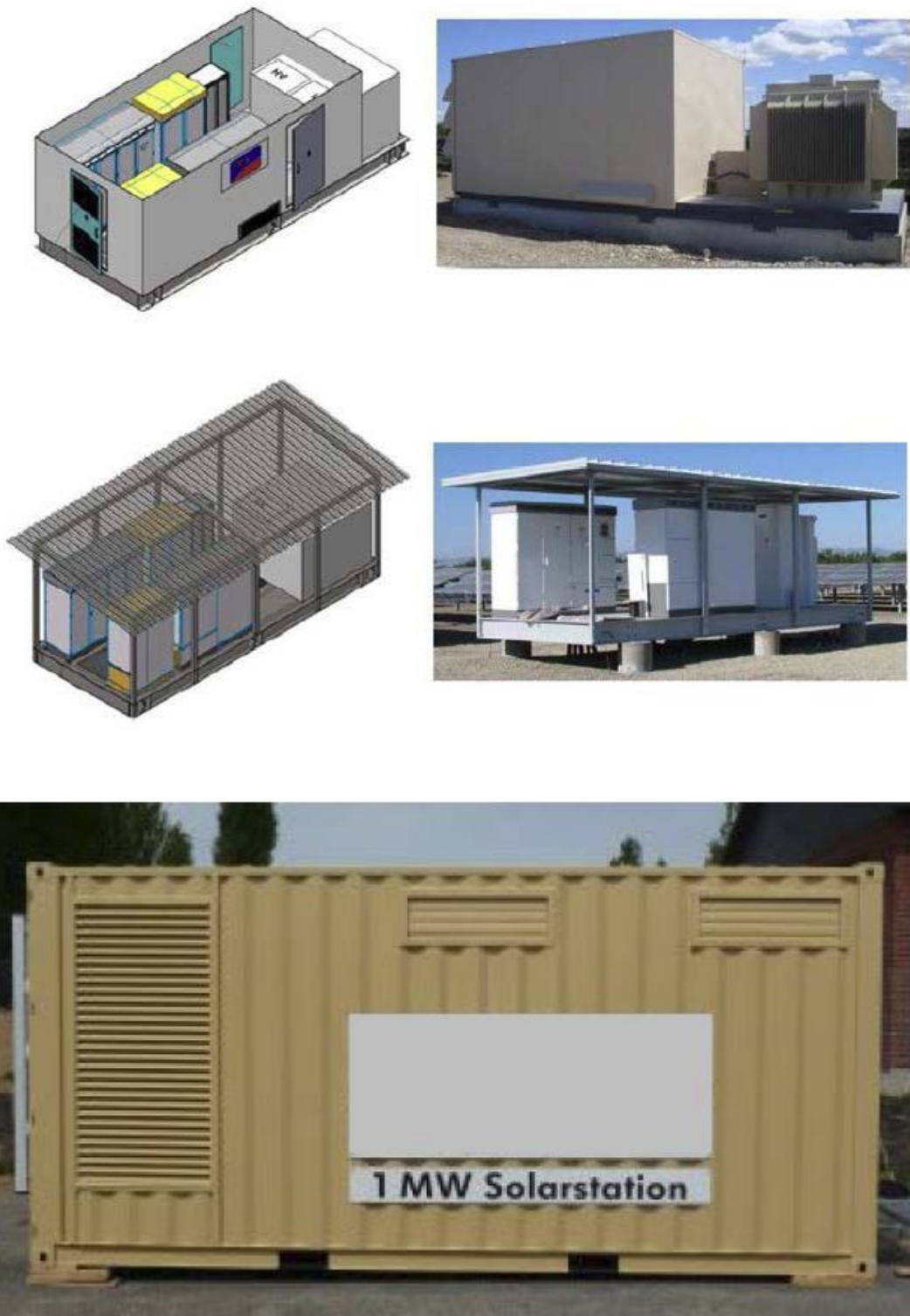
Figure 3-12. Representative Examples of Typical Inverter Stations
