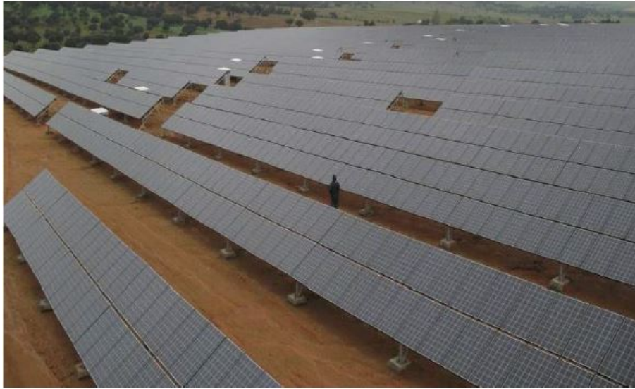
Typical Fixed-Tilt Solar Panel Rows
