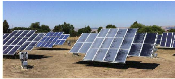
Typical Dual-Axis Tracking Solar Panels
