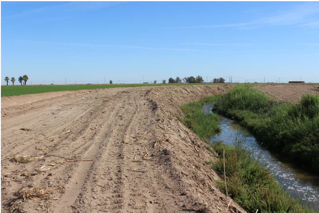
Photo 30: Looking north from the southeast corner subject site 3.
