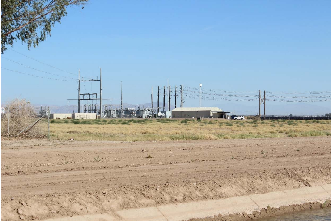
Photo 7: Looking northwest from the southwest corner of subject site 1 at the neighboring solar site substation and control building.
