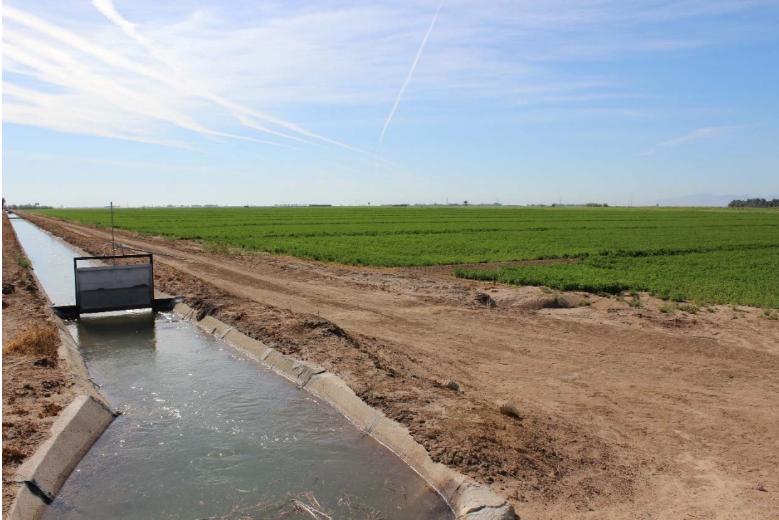
Photo 21: Looking southeast from the middle of sites 1 & 3.
