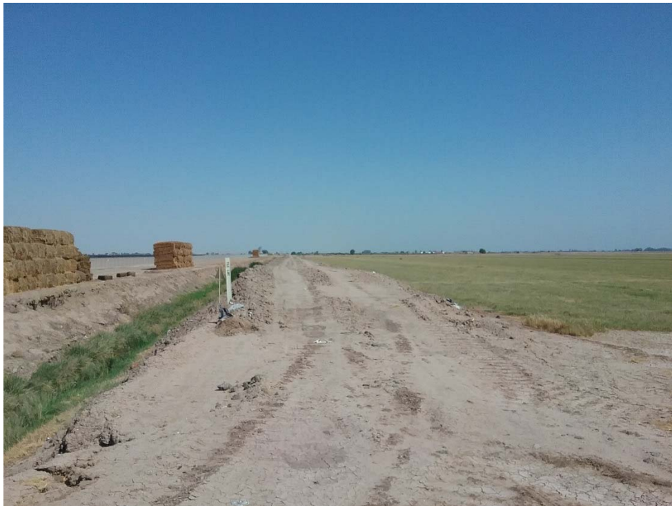
Photo 38: Looking north from the southwest boundary of site 4.
