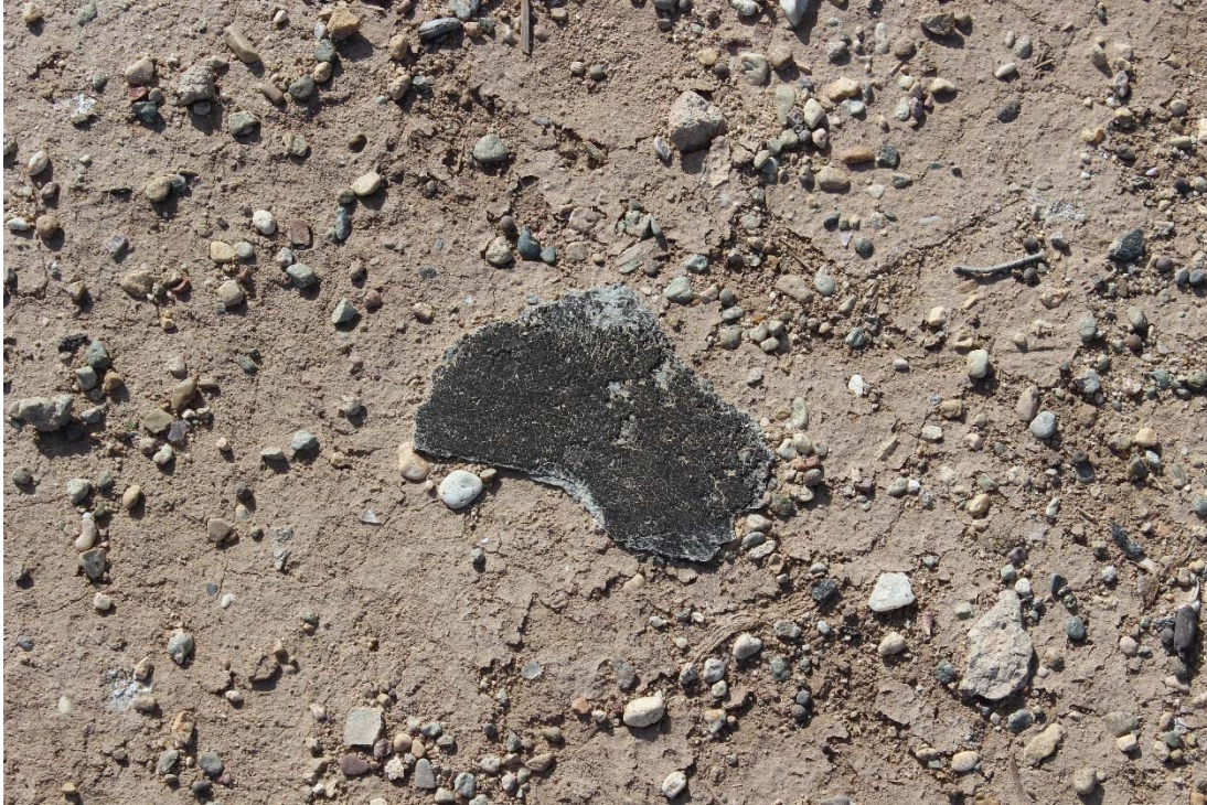
Photo 9: Looking roof shingles blown off structure at property south of subject site.
