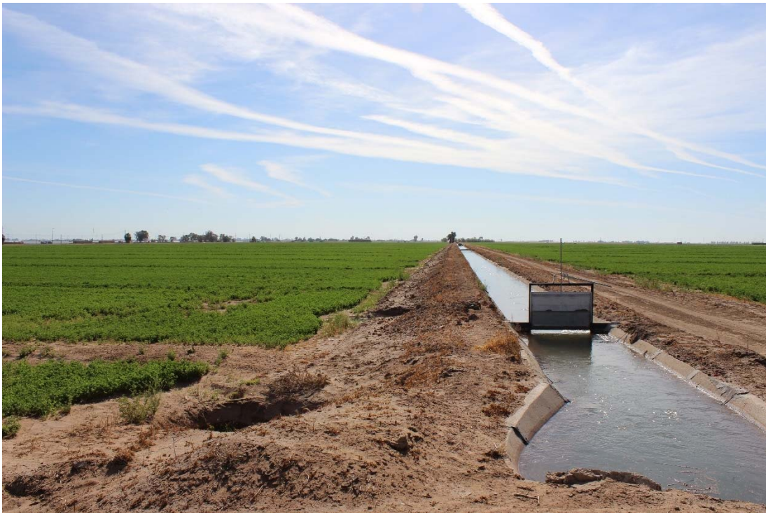
Photo 20: Looking east from the middle of sites 1 & 3.
