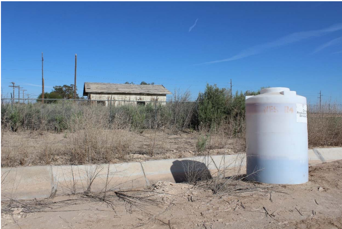
Photo 10: Looking at chemical tank used to apply fertilizer to irrigation water found at south end of subject site 1.
