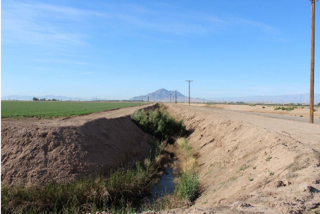
Photo 1: Looking south from the northwest corner of the subject site.
