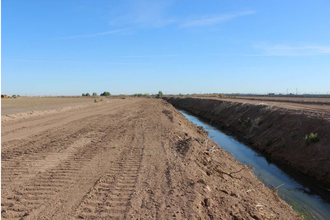
Photo 9: Looking north from the southeast corner of the subject site.
