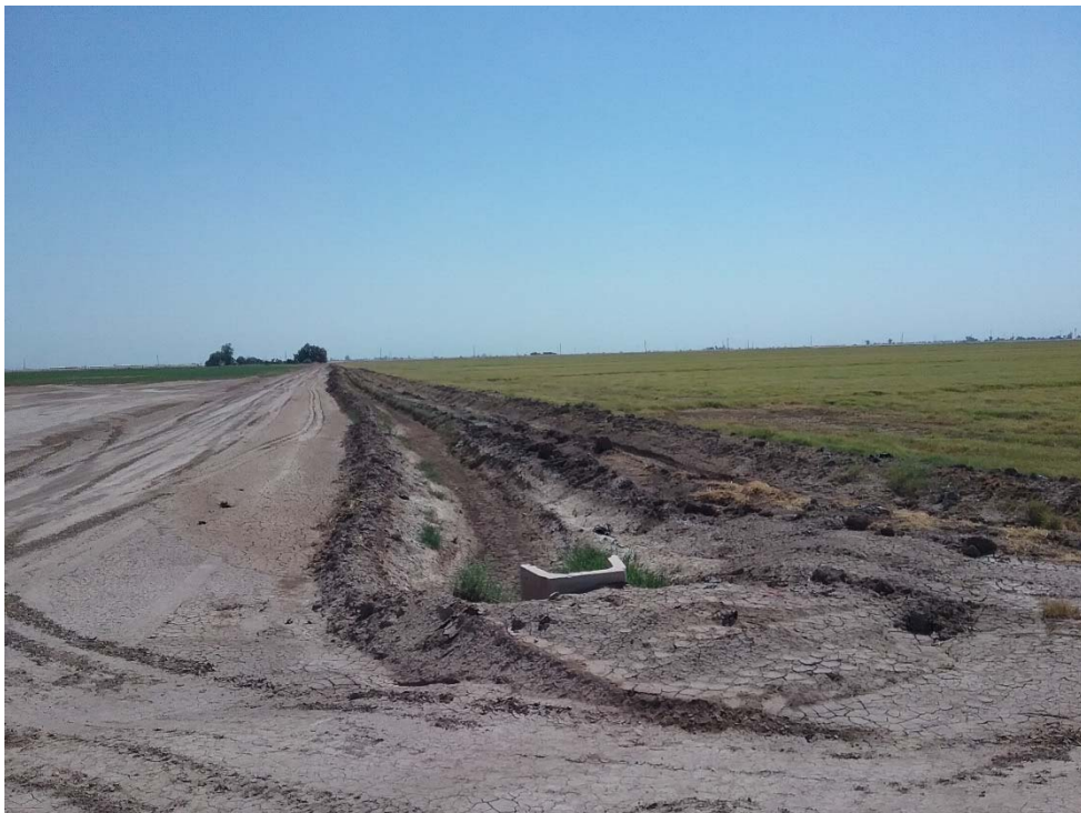
Photo 8: Looking east along the northern boundary of Site 1 (SE).
