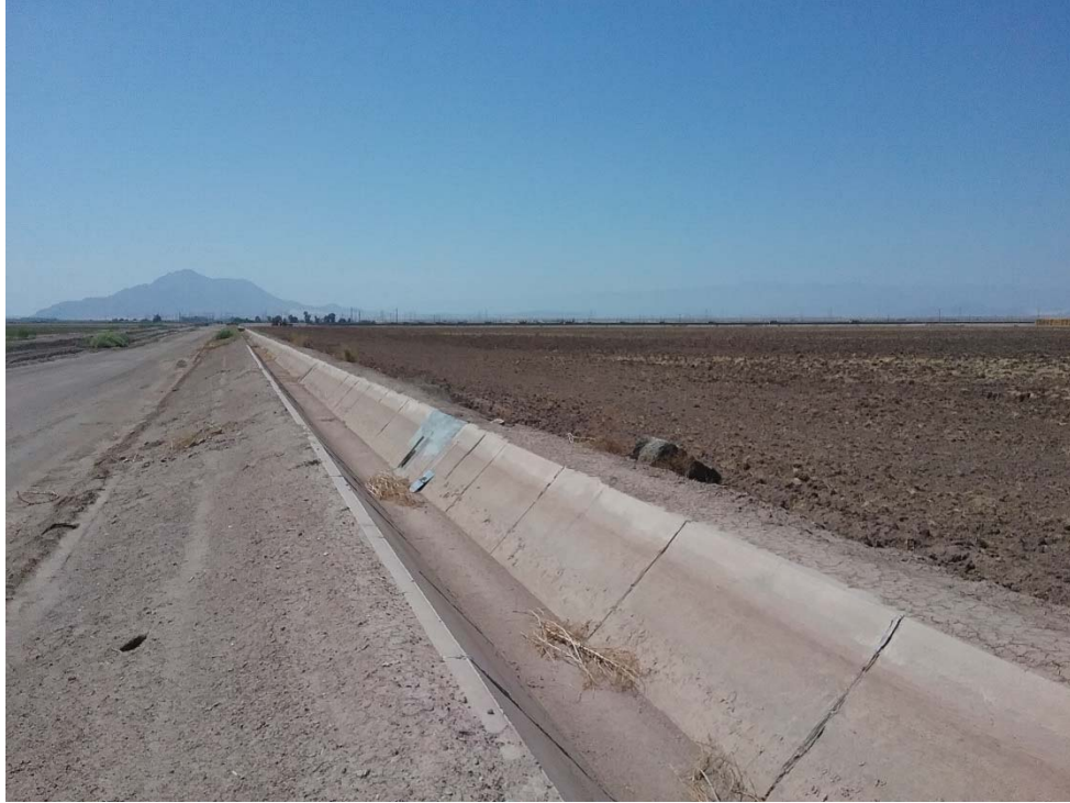
Photo 13: Looking south from the northeast corner of Site 2 (NW).
