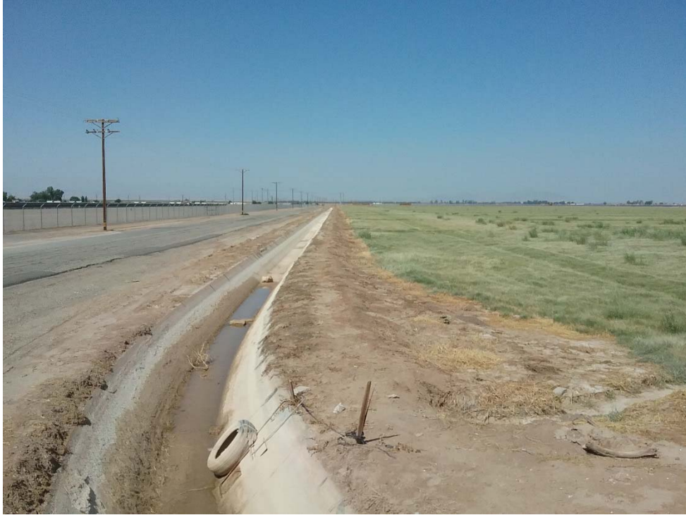
Photo 1: Looking north along the western boundary of Site 1 (SE).
