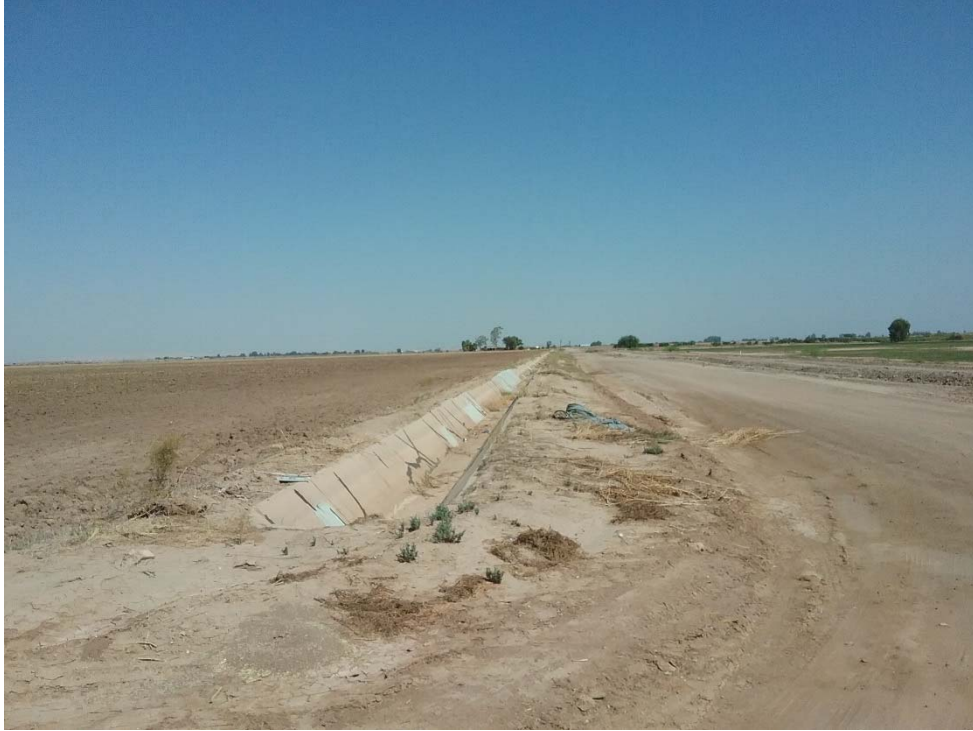
Photo 11: Looking north along the eastern boundary of Site 2 (NW).
