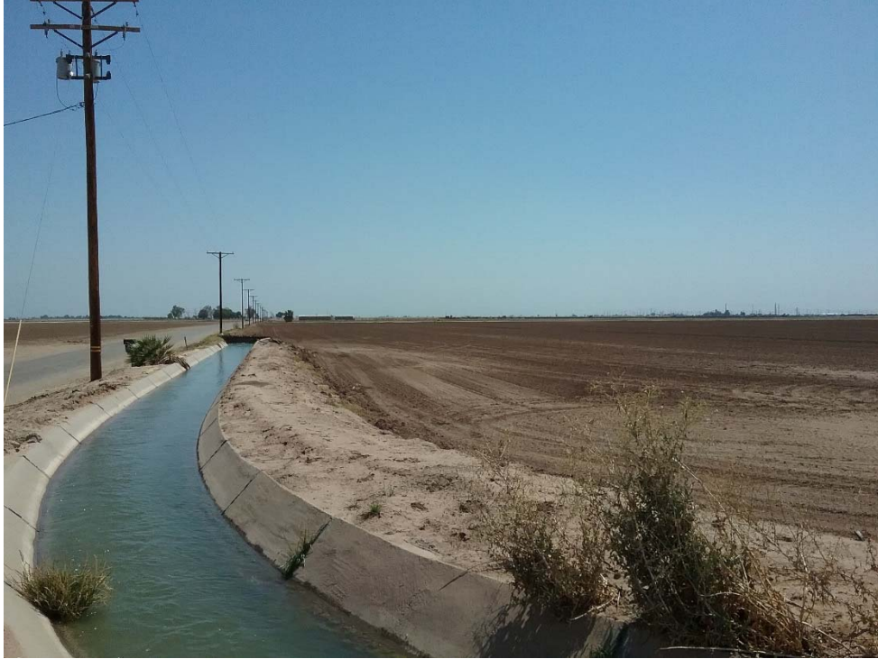
Photo 31: Looking east from the northwest corner of Section 4.
