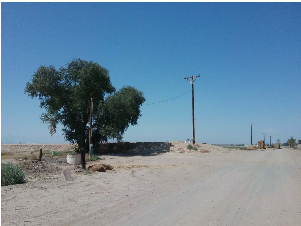
Photo 4: Looking at the drain pump and transformer located along the middle of the northern boundary of Section 1.
