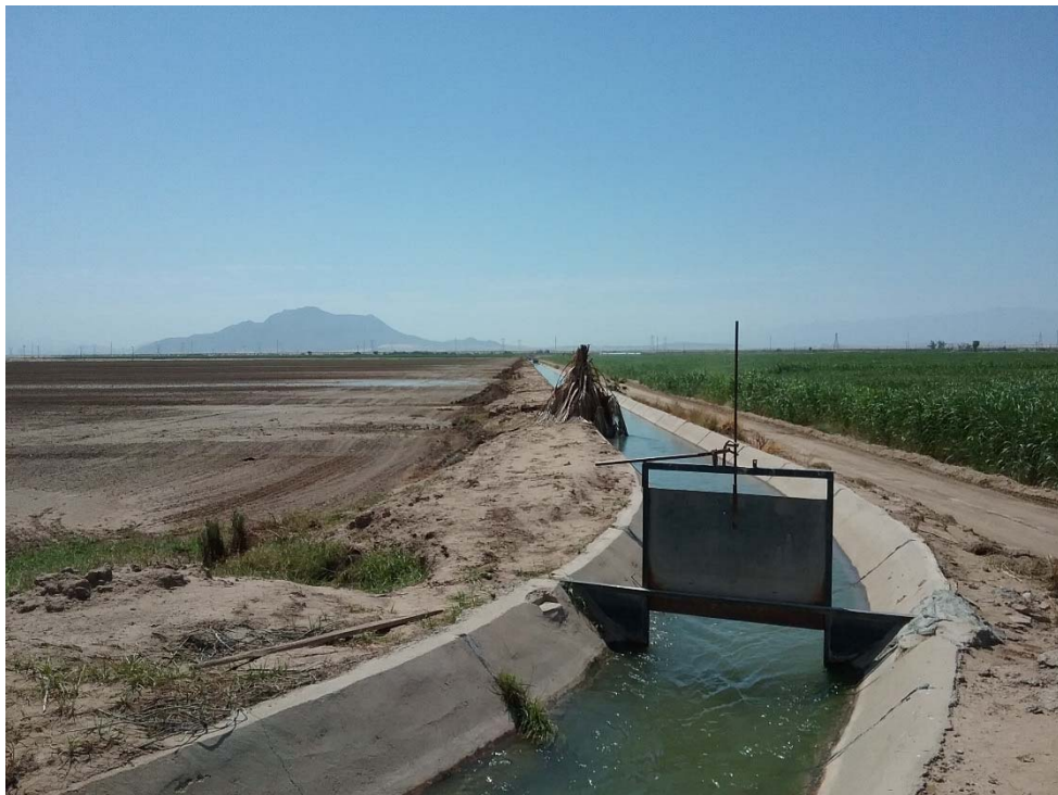
Photo 30: Looking south from the northwest corner of Section 4.
