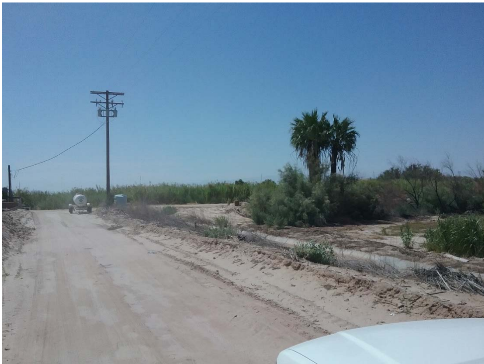
Photo 24: Looking at the southeast corner of Section 5 at the transformer mounted on IID power pole.
