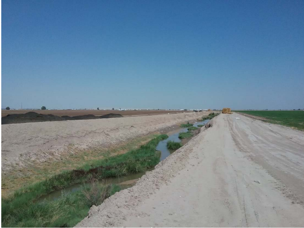
Photo 13: Looking northwest across the Dixie Drain Three within Section 2.
