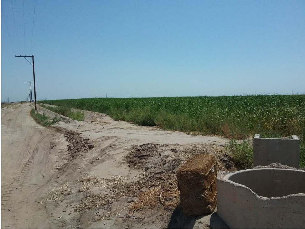
Photo 27: Looking east from the northwest corner of Section 5.
