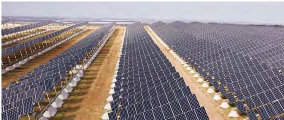
Typical Single-axis Tracking Solar Panel Rows
