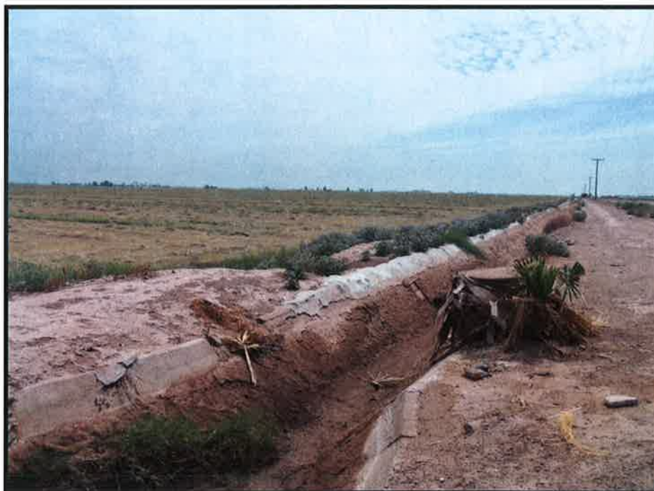
Photo 21: Looking east along the southern boundary of the site.
