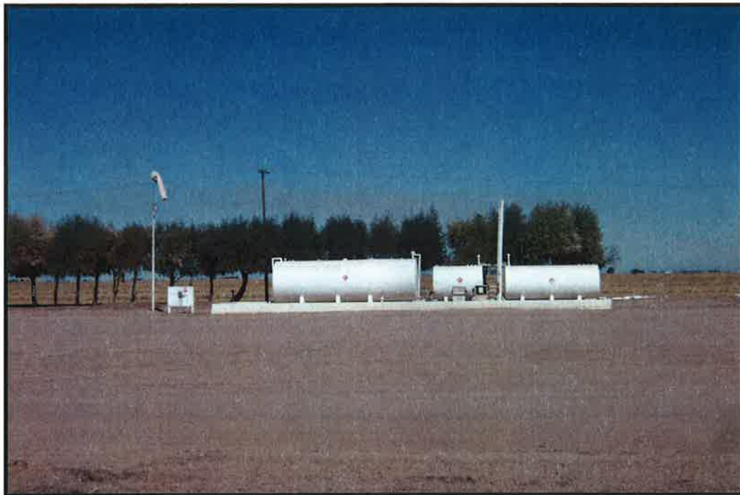
Photo 15: Gasoline storage tanks within a concrete containment area.
