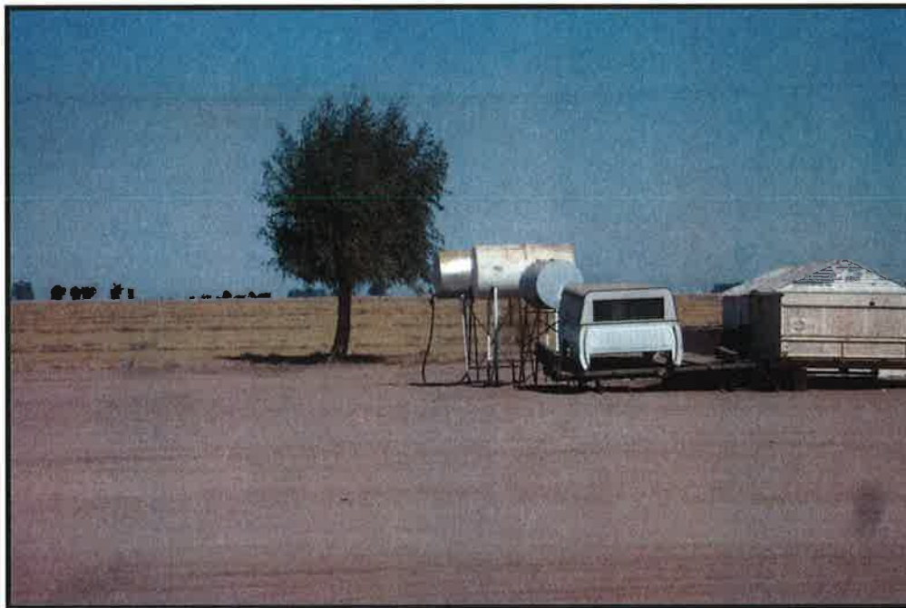
Photo 14: Above ground storage tanks on the native soils at the crop dusting facility.
