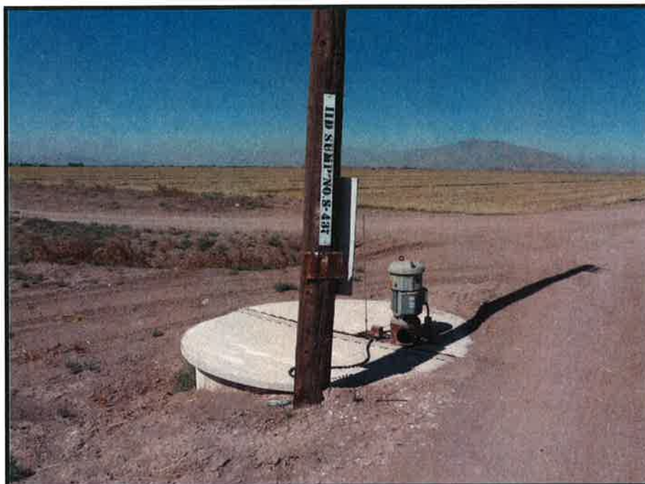
Photo 4: IID sump located at the central northern boundary of Section II.
