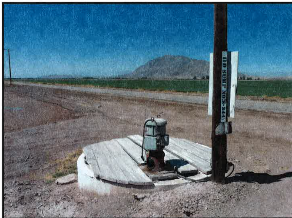
Photo 2: IID sump on the northwest corner of Section IV.
