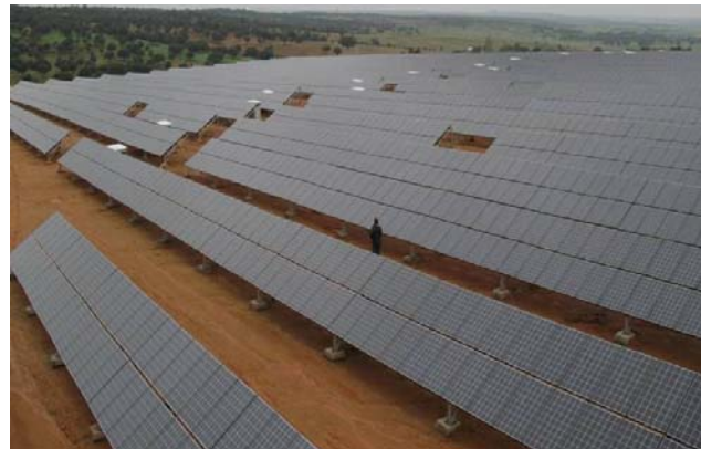
Typical fixed-tilt solar panel rows
