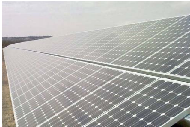
Fixed-tilt solar panels
