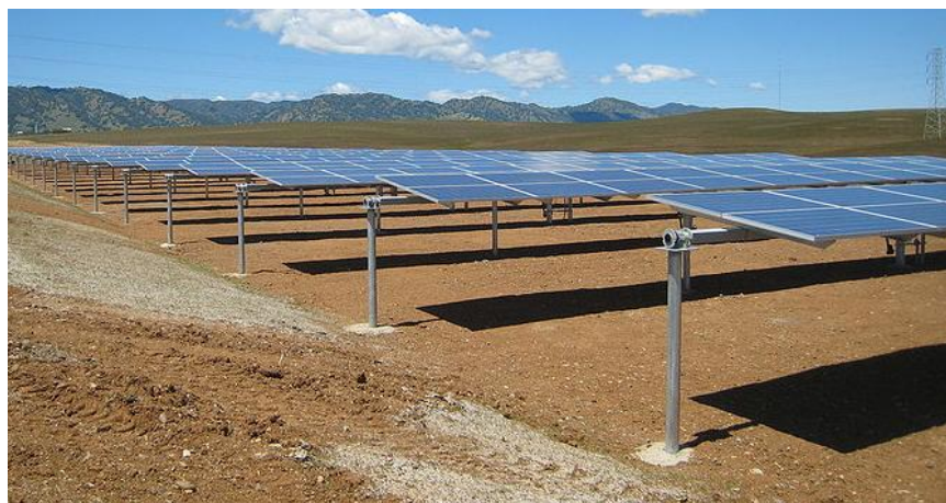
Typical single-axis tracking solar panel rows
