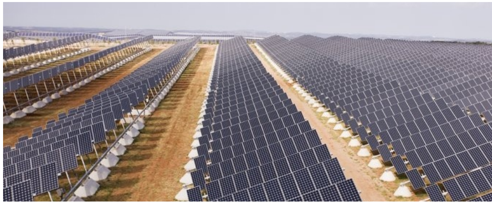
Typical single-axis tracking solar panel rows
