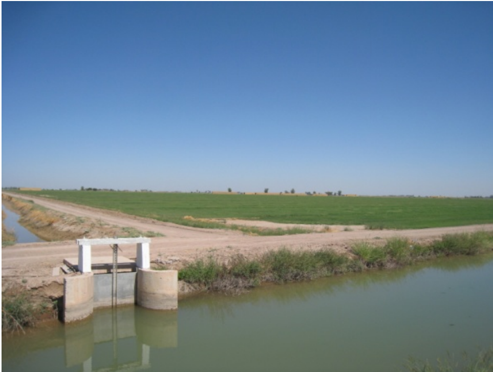
Figure 8: Parcel I, location #4 looking northeast
