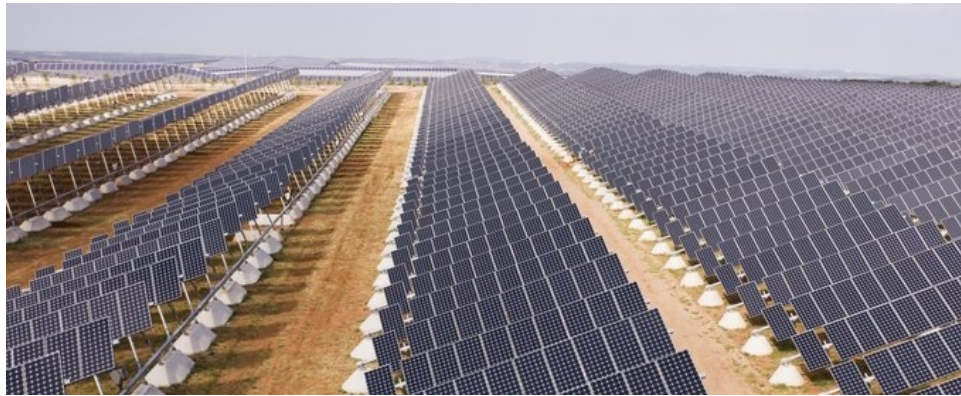
Typical single-axis tracking solar panel rows
