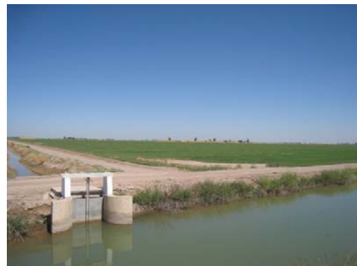
Parcel I, #4 Looking NE
