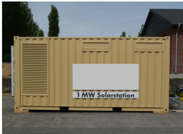
Typical Inverter Container
