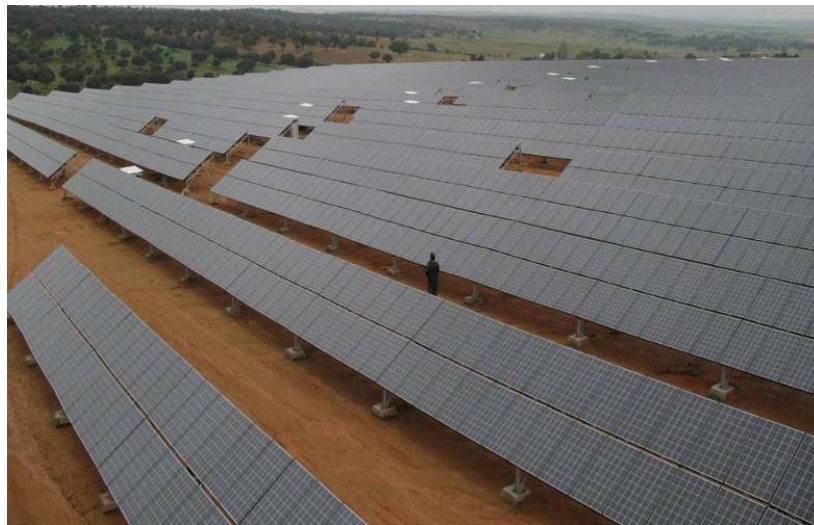
Typical fixed-tilt solar panel rows
