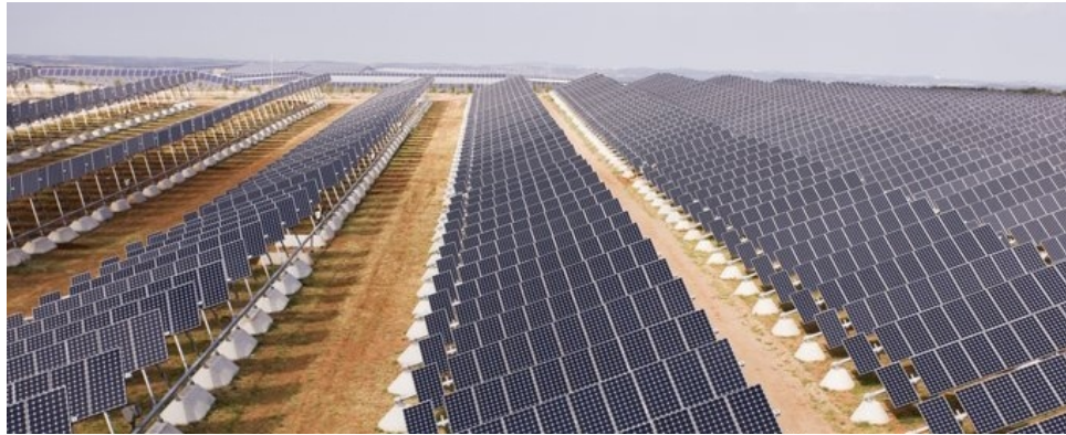
Typical single-axis tracking solar panel rows
