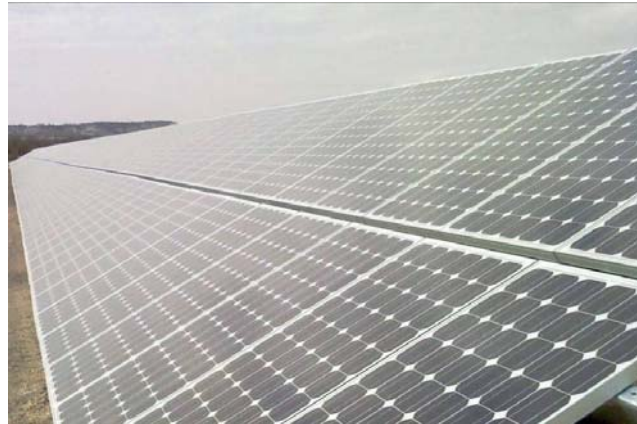
Fixed-tilt solar panels
