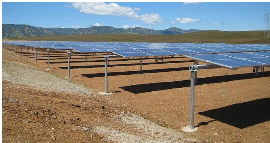
Typical single-axis tracking solar panel rows
