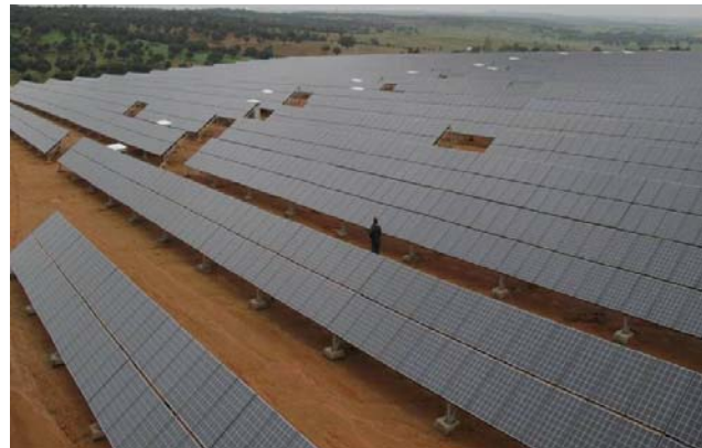
Typical fixed-tilt solar panel rows
