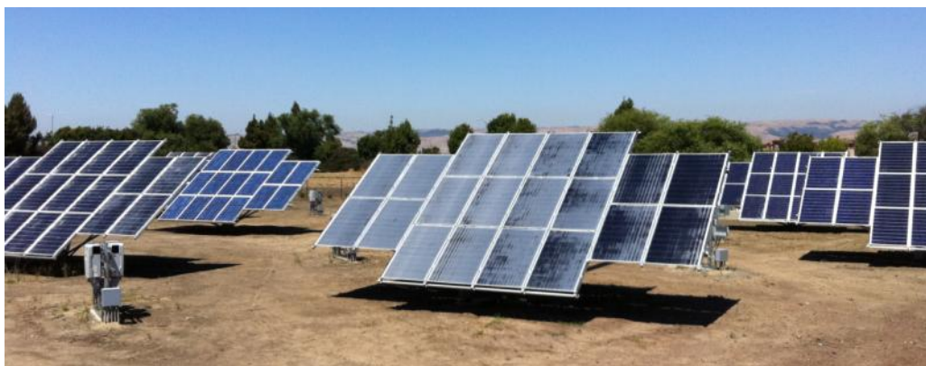
Typical azimuth tracking solar panel rows
