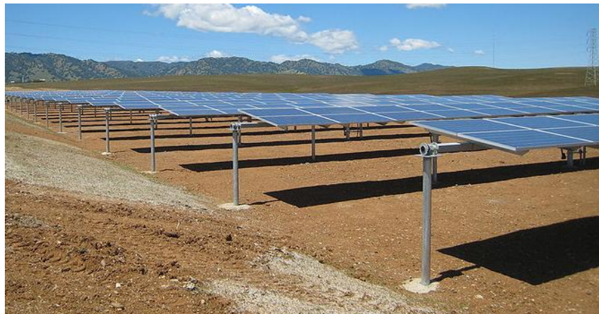
Typical single-axis tracking solar panel rows
