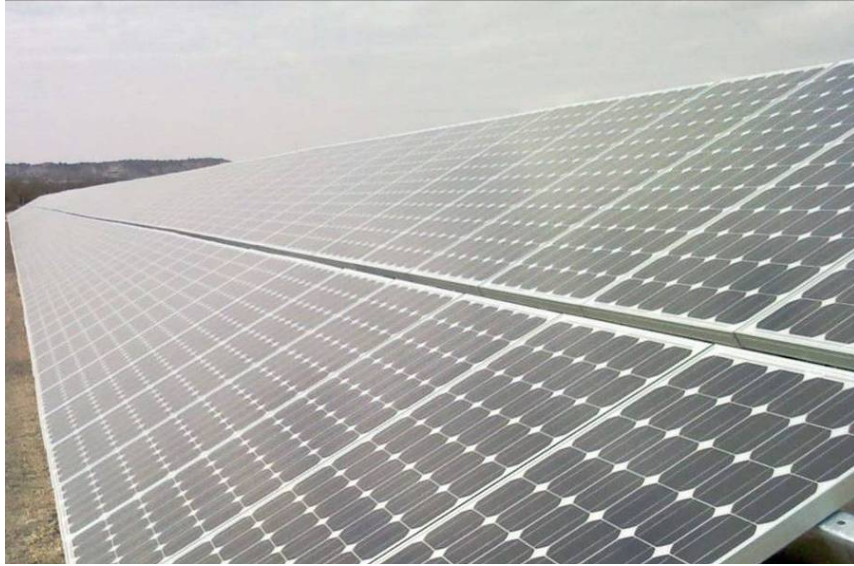
Fixed-tilt solar panels
