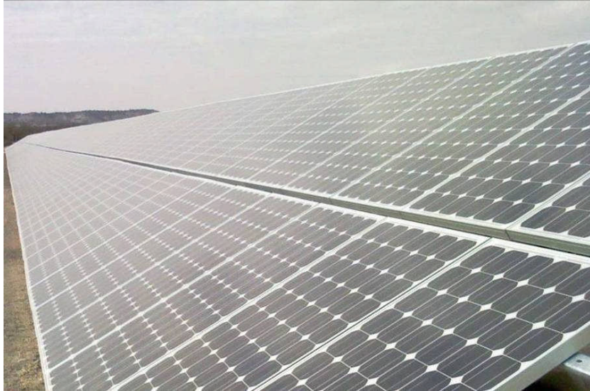
Fixed-tilt solar panels
