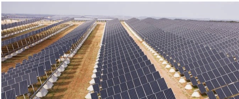
Typical single-axis tracking solar panel rows
