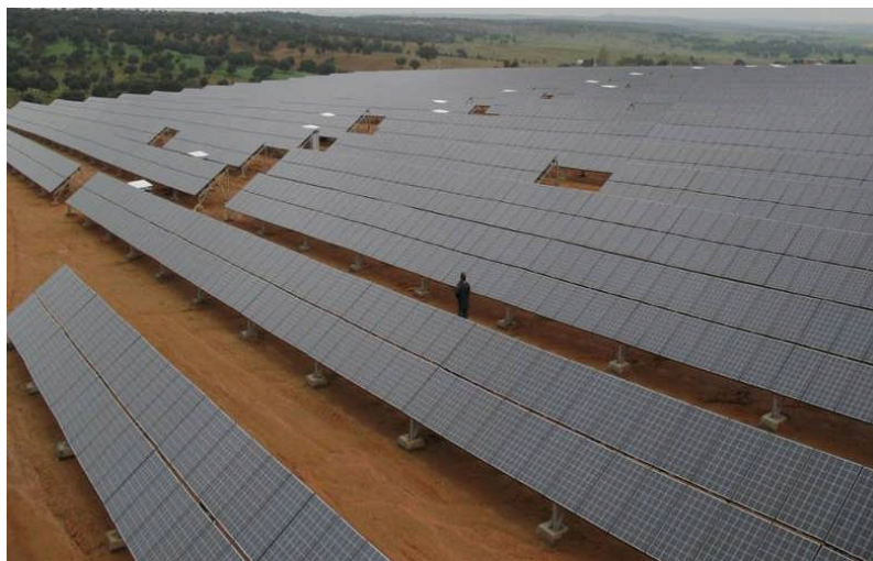
Typical fixed-tilt solar panel rows
