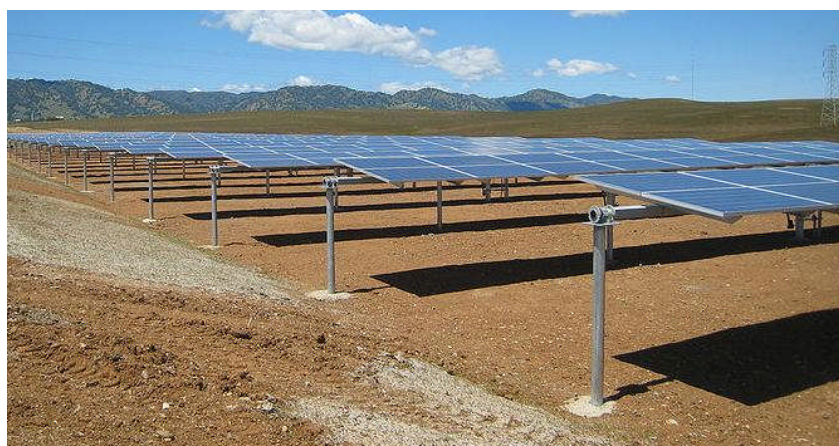
Typical single-axis tracking solar panel rows
