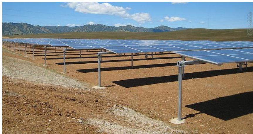
Typical single-axis tracking solar panel rows
