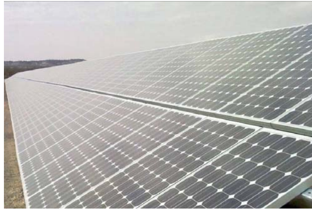
Fixed-tilt solar panels
