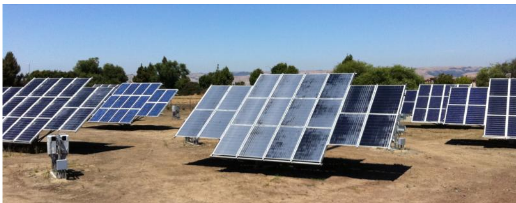
Typical azimuth tracking solar panel rows
