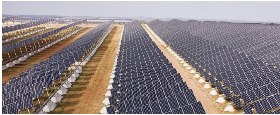
Typical single-axis tracking solar panel rows
