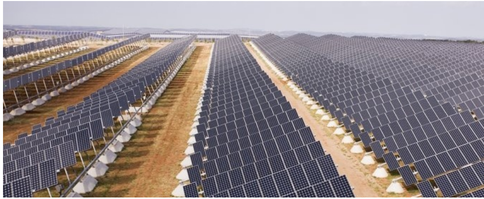
Typical single-axis tracking solar panel rows
