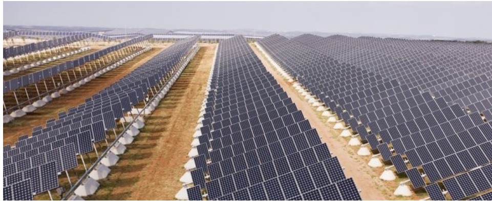
Typical single-axis tracking solar panel rows
