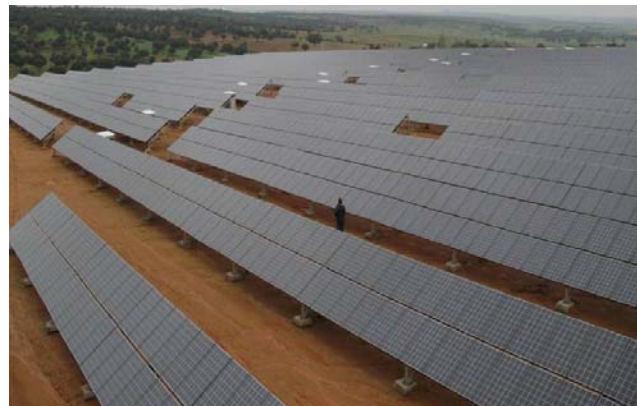
Typical fixed-tilt solar panel rows
