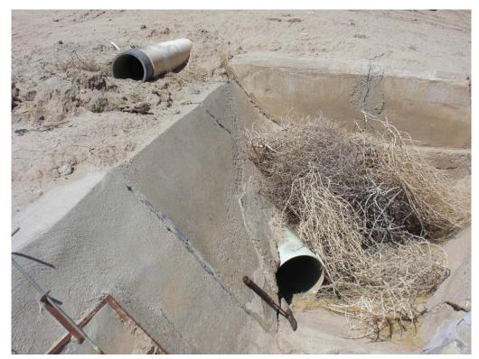
Photograph 15: Outcropping of PVC Pipeline and Concrete Irrigation Structures on the Property
