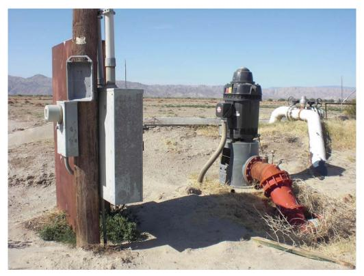
Photograph 13: Water Well #4 and Irrigation Structure Interconnection on the Property
