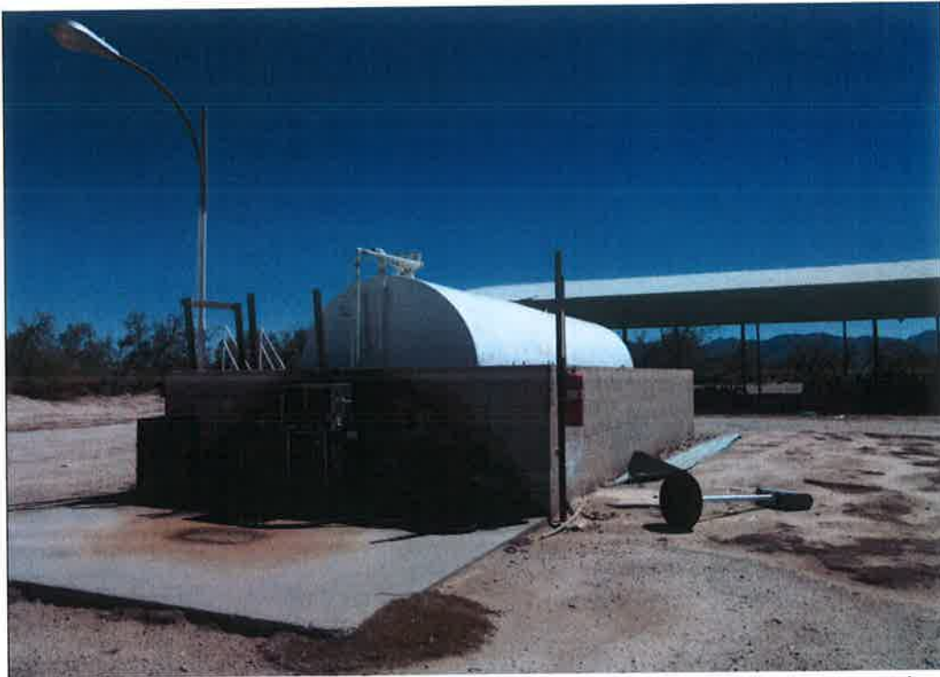
Photo 4: Looking at fuel tank/pump that is located on the west side of Section 1.
