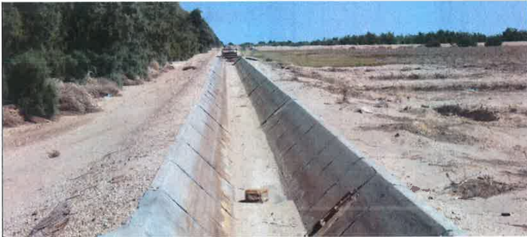
Photo 17: Looking east from the north side of Section 4.
