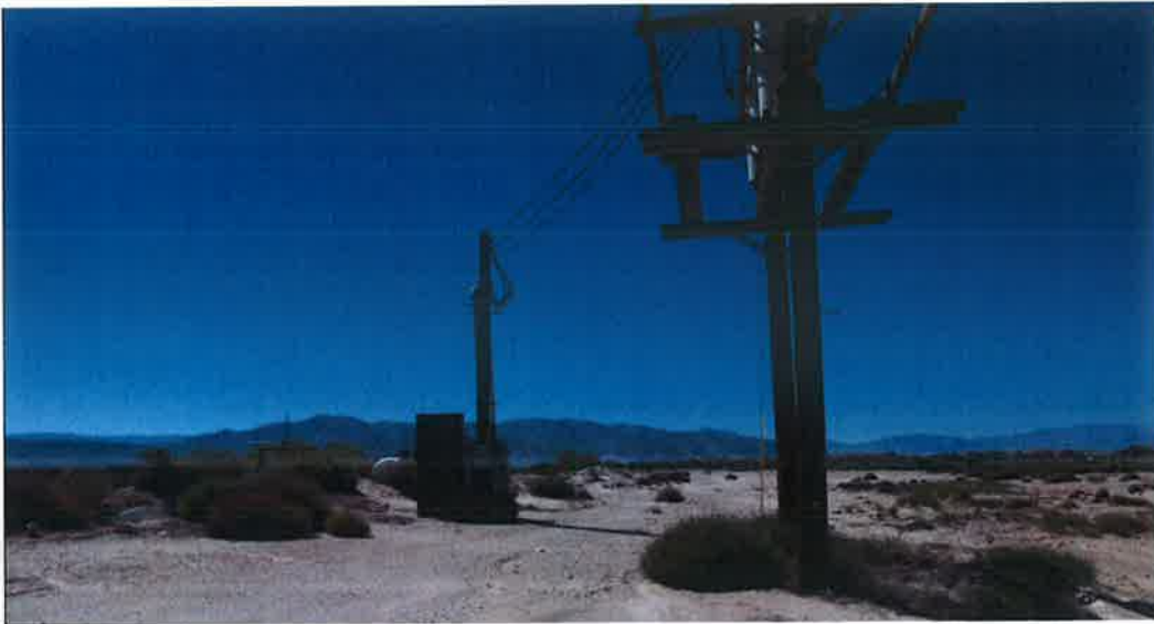
Photo 11: Looking west from the southwest corner of Section 2.
