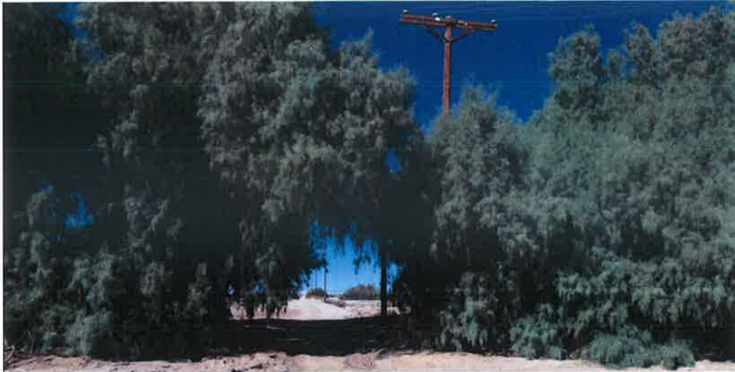
Photo 21: Looking north from the north side of Section 3 at the power lines that feed items in Photo 20.
