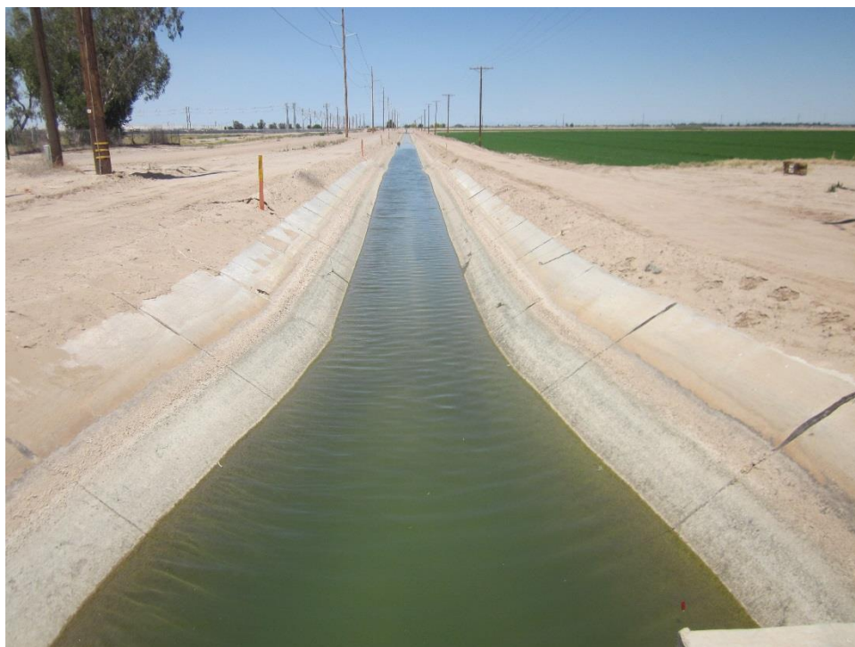
Figure 7. P-13-012689 Fern Canal, facing north.
