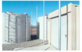
Typical system configuration with two 10,000-gallon tanks and plant in building The Project may also utilize an additional 10,000 gallon storage tank or tanks to store treated water for sanitary uses. Potable water will be trucked to the site.
