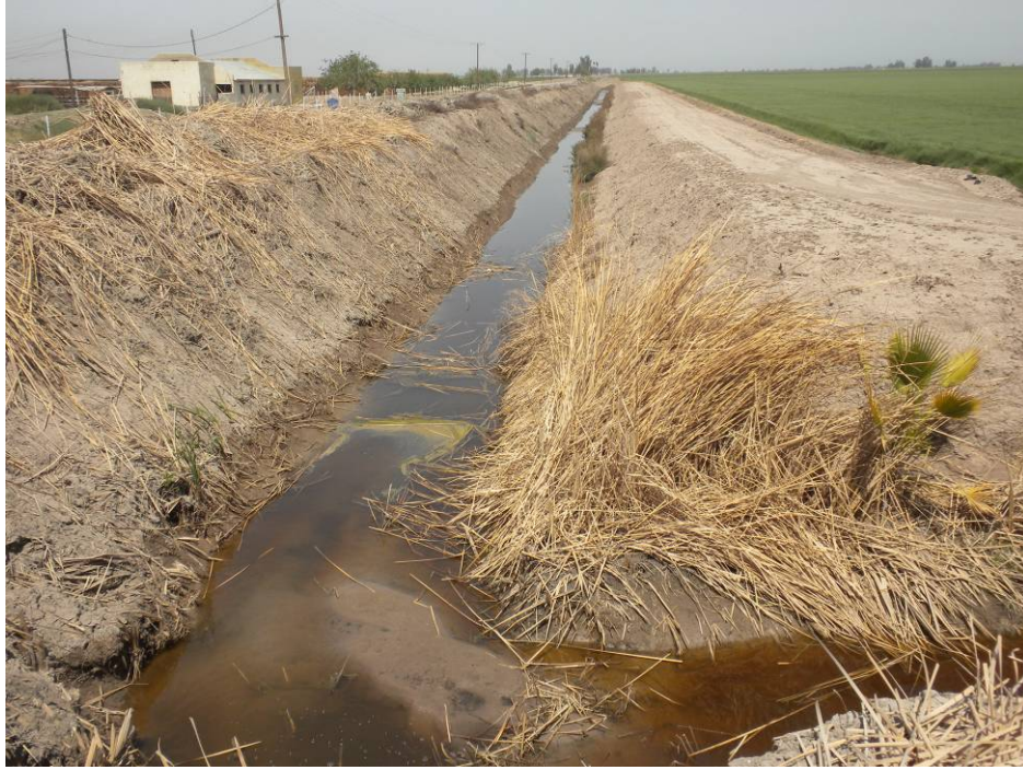
Evidence of removal of emergent vegetation through maintenance activities from dirt-lined channel.
